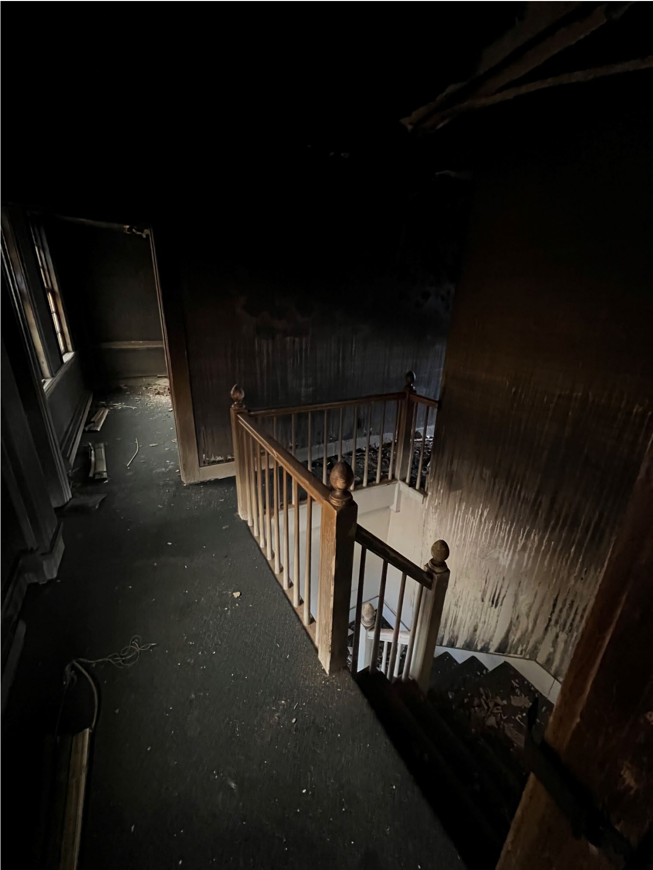
Interior Fire Damage
