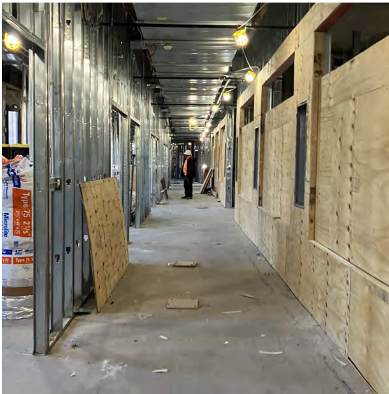
Plywood Installed Along New Main Corridor
