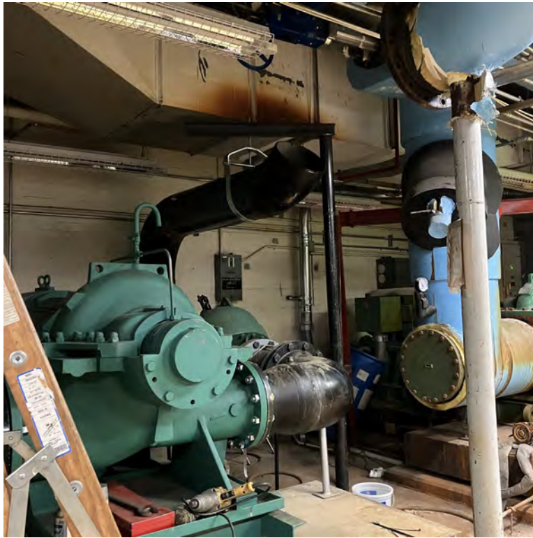
Chilled Water Pump #4 Pipe Installation
