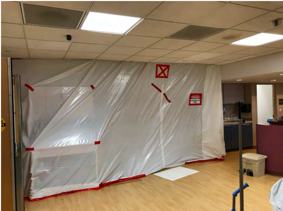
View of Temporary Barrier at Nurse's Station
