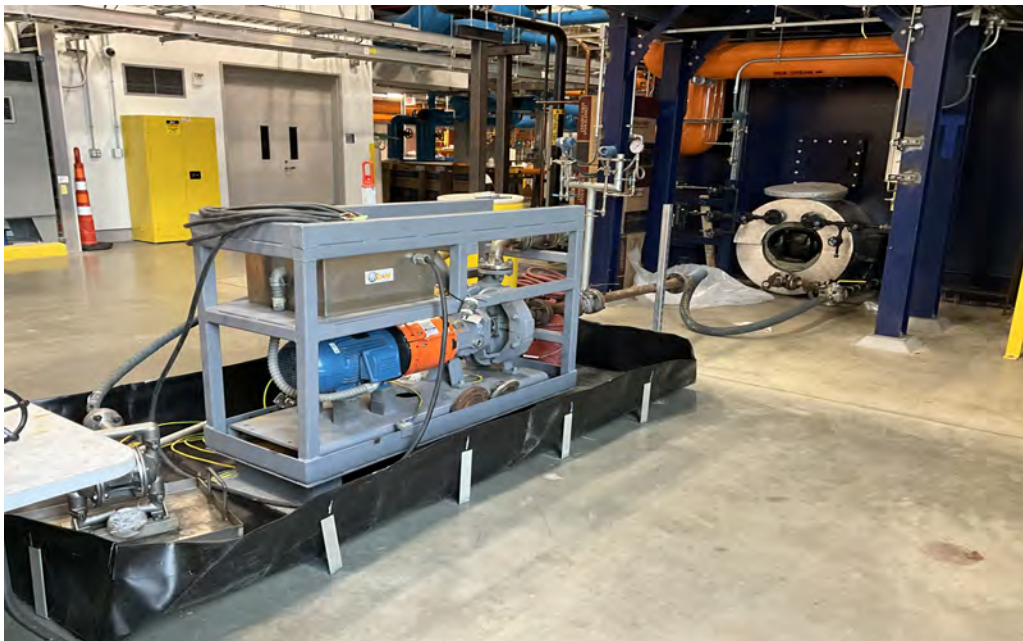
Temporary equipment set up for boil out process
