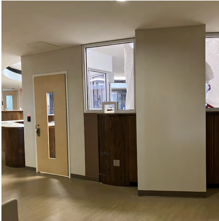
New Nurse Station Enclosure with Pass Through Opening
