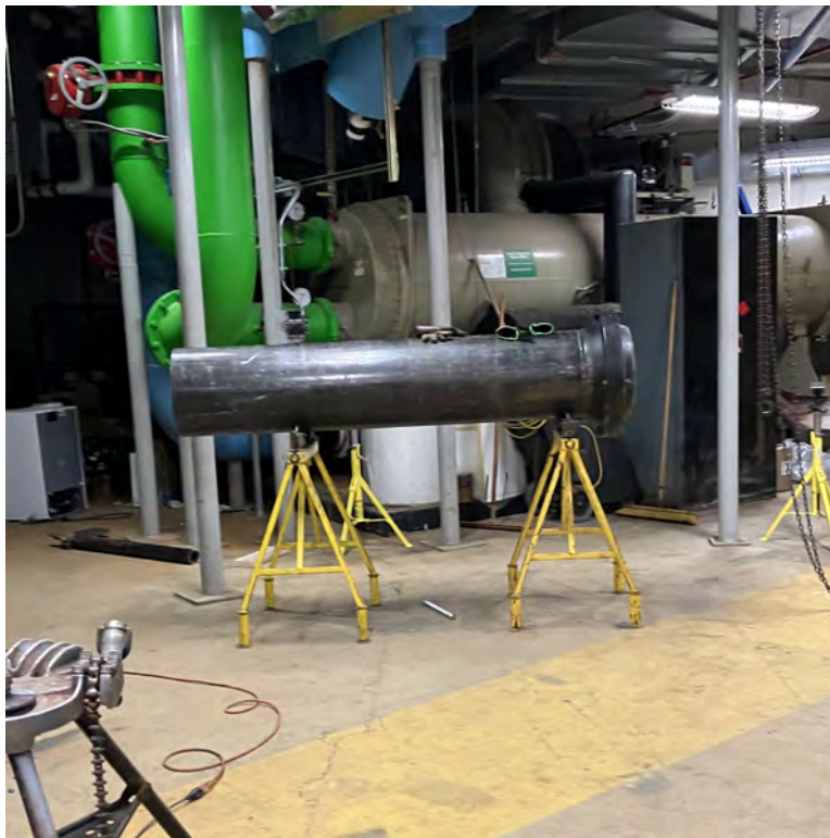
Chilled Water Pump #4 Pipe Preparation
