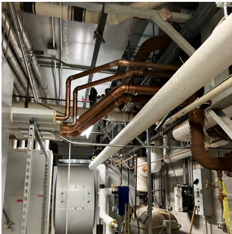
New 3" & 1 1/2" Hot Water Pipe Entering Sub-basement Corridor
