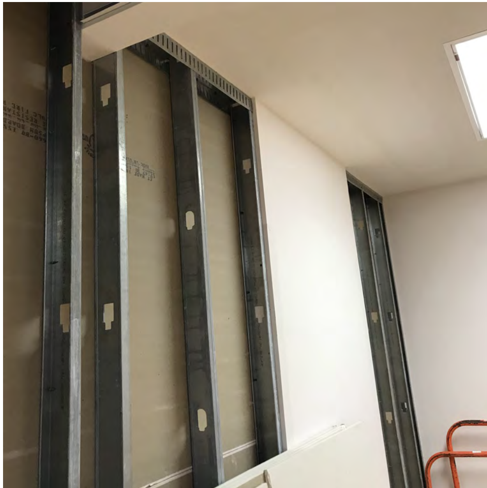
View of New Demising Wall Between Endo/GI and Hyperbaric Chamber Room
