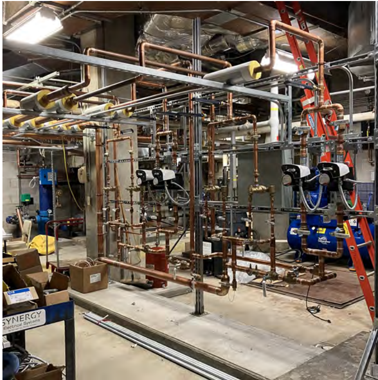
New Circulation Pump Station & Steam Hot Water Heater
