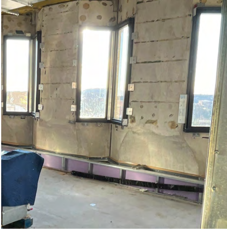
New Windows and 2 Hour Shaft Wall along Perimeter
