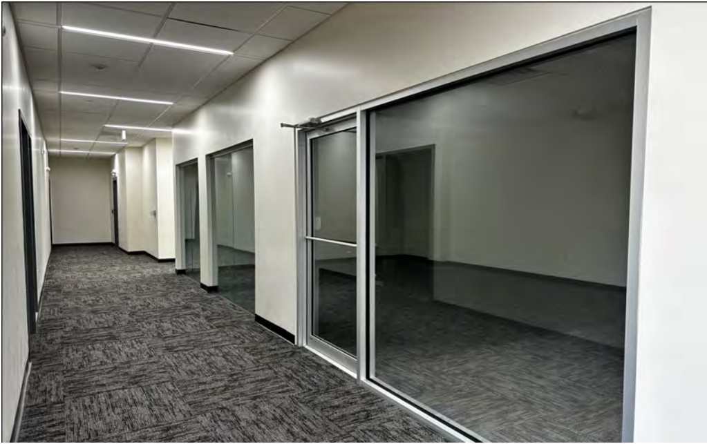
Waterbury progress photo interior offices.
