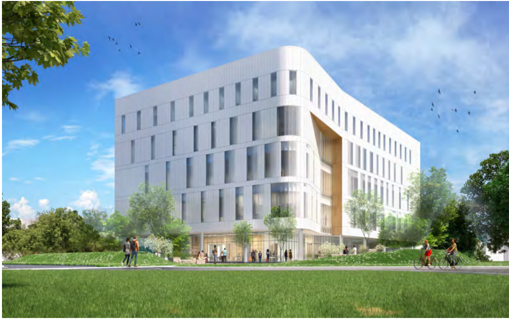
Nursing Building Exterior - Southwest Elevation
