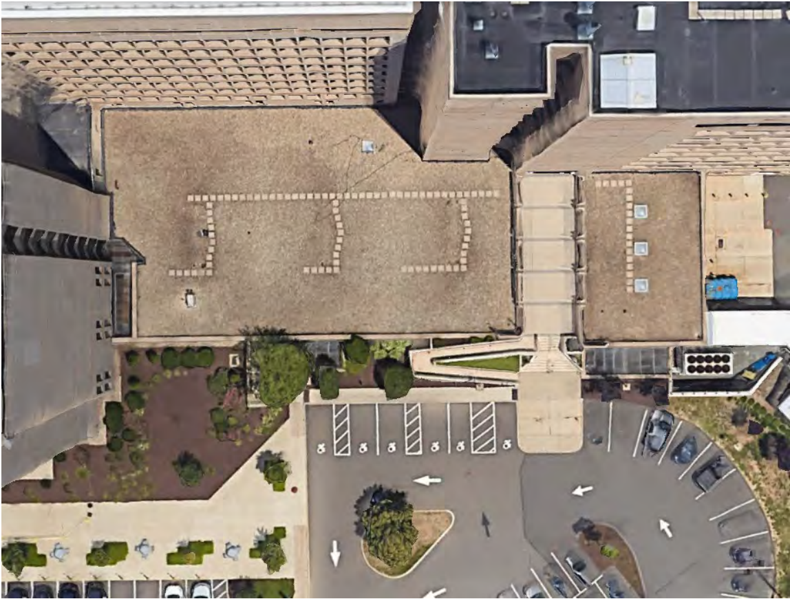
Existing Building K Roof
