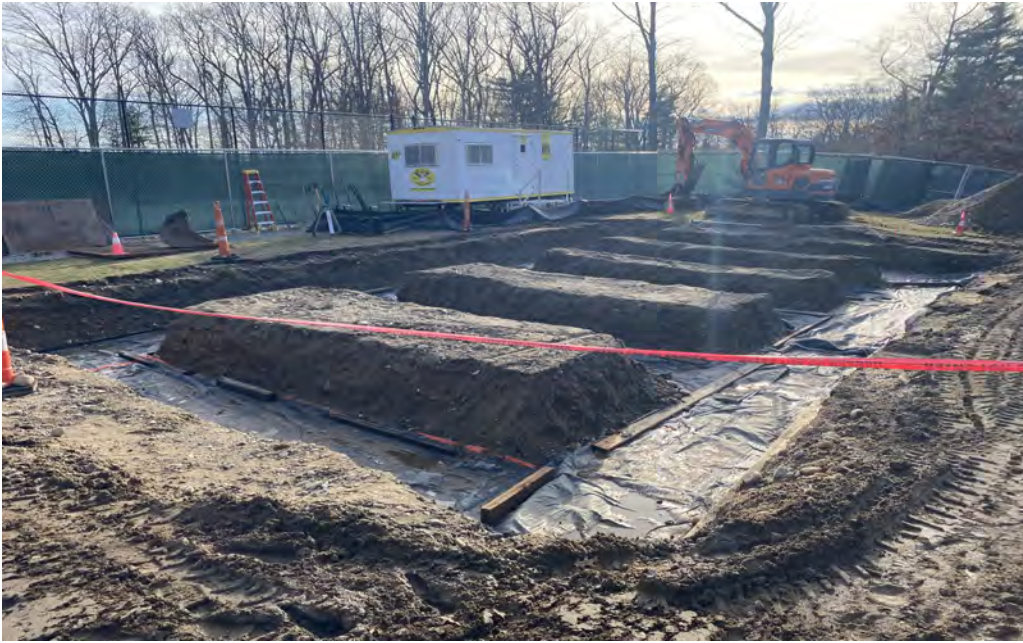
Foundation excavation prepared for forms and concrete.
