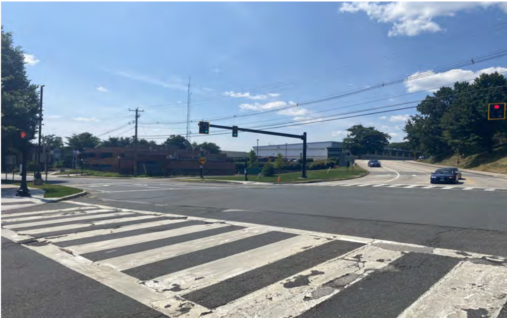
NW corner of NER and Discovery Dr - New Signals in Operation
