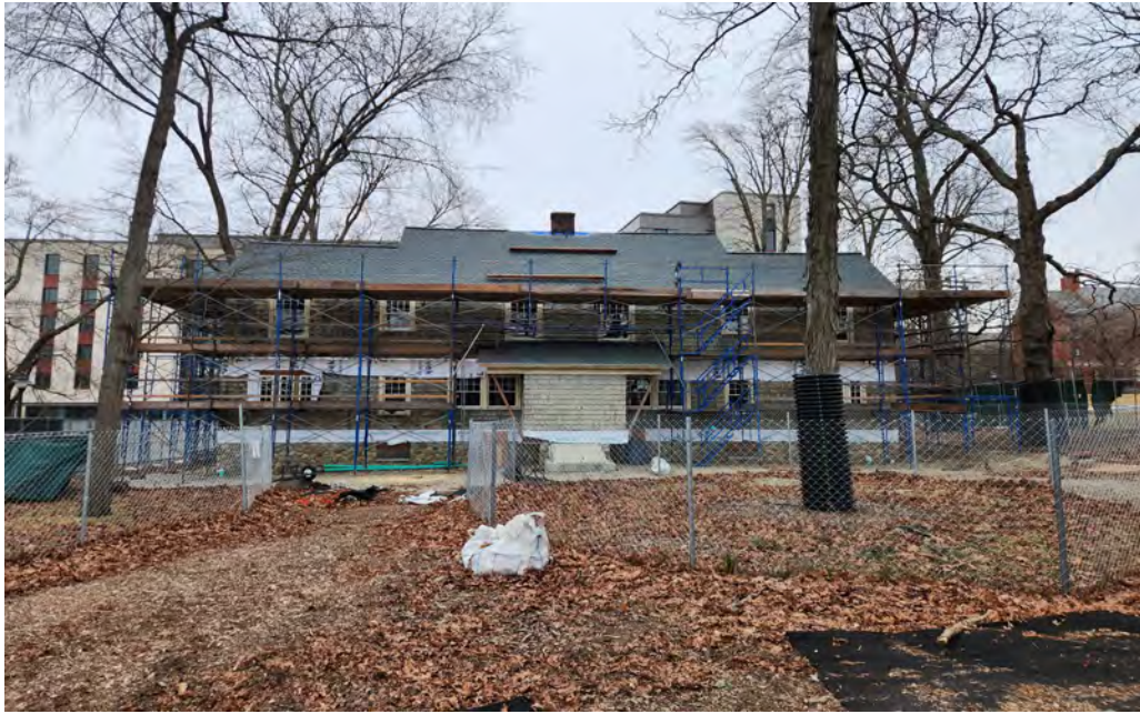
Roof and Facade progress
