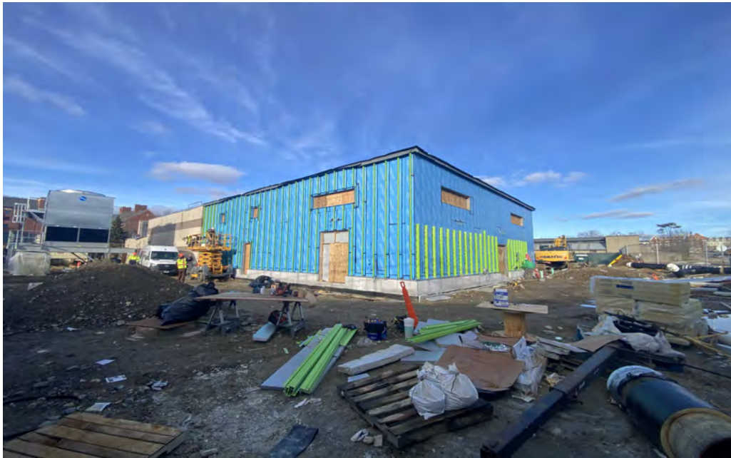
Building weather tight and finishes starting
