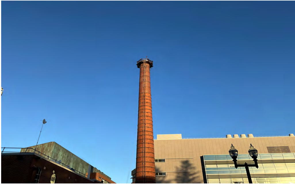
CUP chimney with ladder to top for gutter installation
