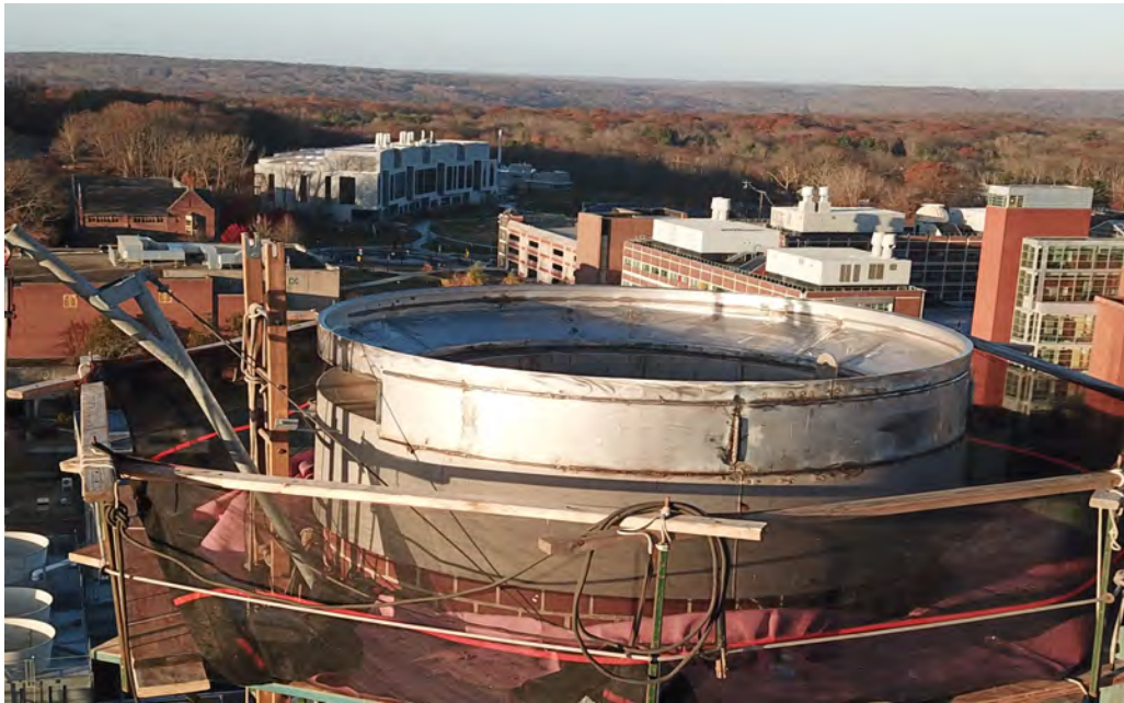
Gutter installation at top of existing CUP chimney
