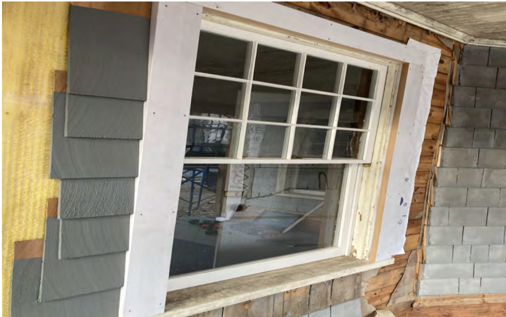
Facade shingles mockup
