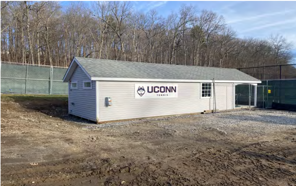
Relocated shed for use during construction
