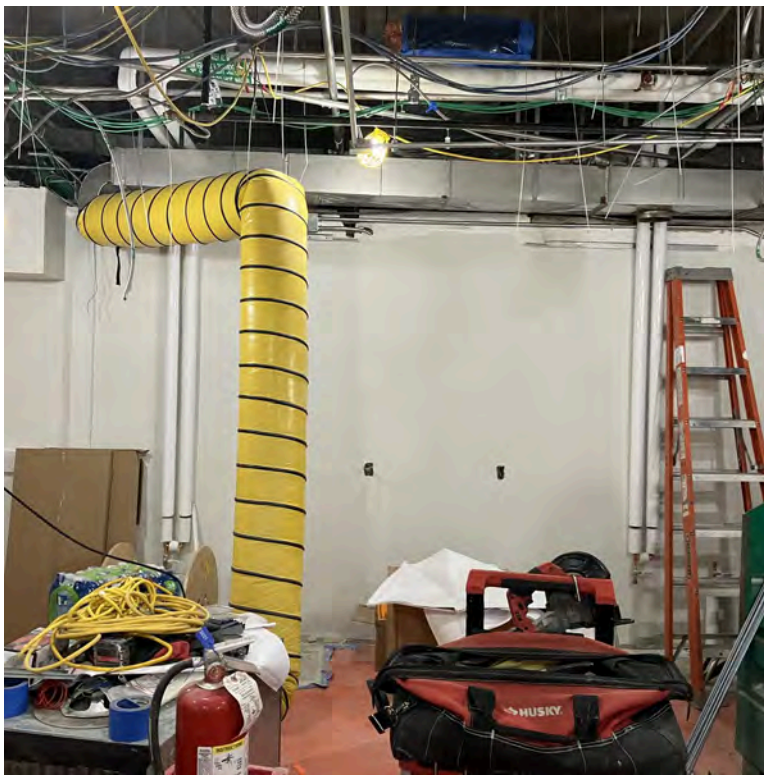
New Ductwork, Plumbing, & Electrical for Crossing Stations
