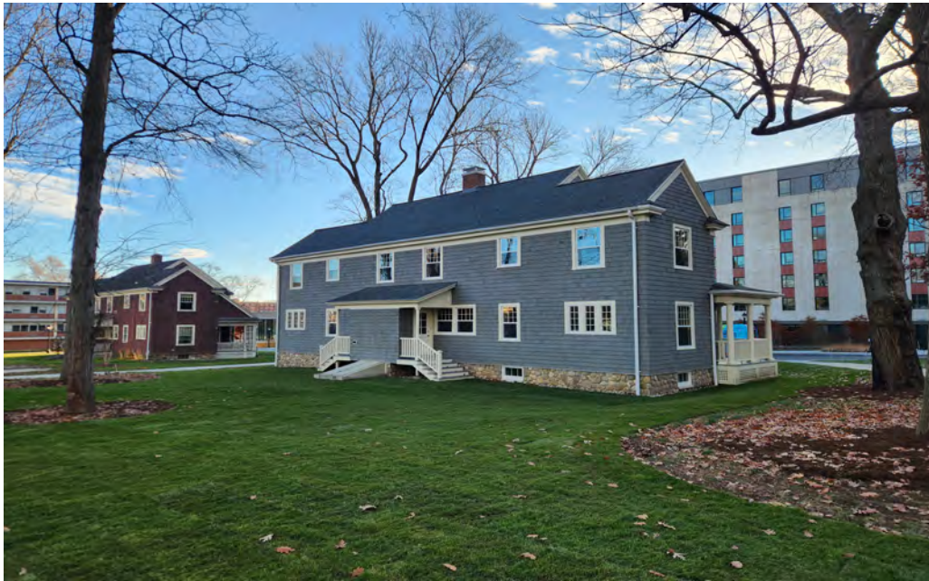
Back entry view
