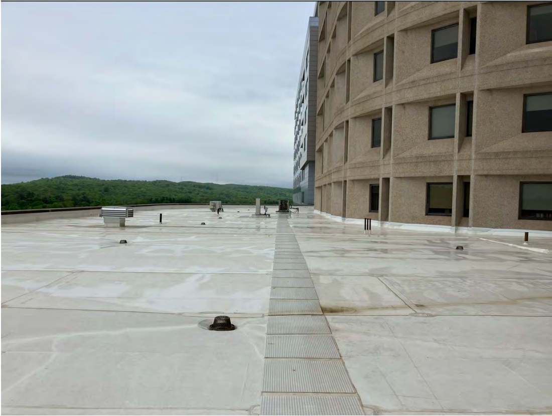
Completed Building F Roof
