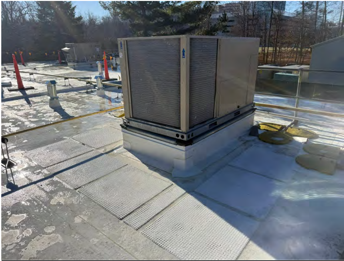
Completed Building M Roof
