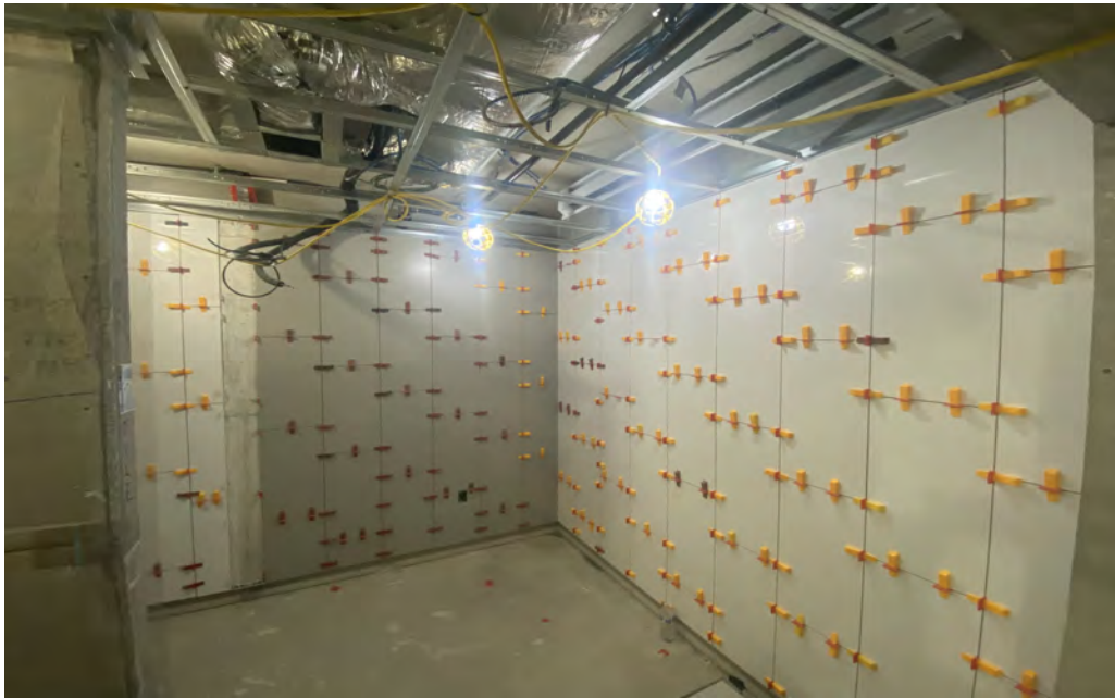
Tile in team bathroom
