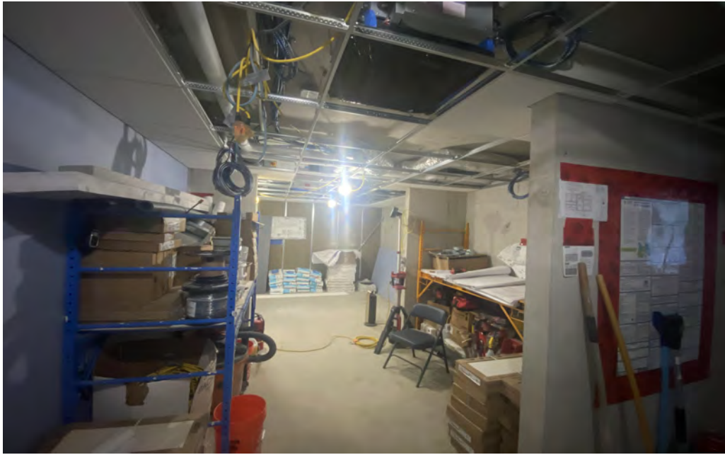
Team locker room with rough MEP complete
