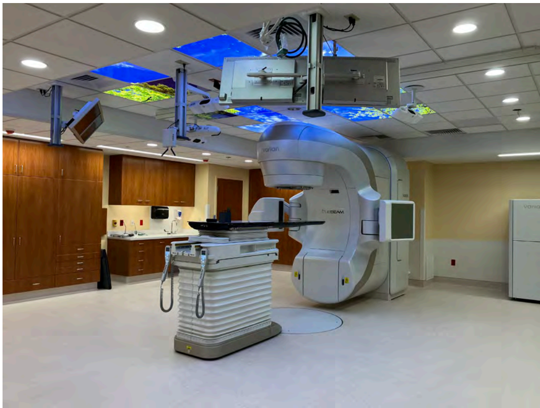
S1868 New LINAC unit
