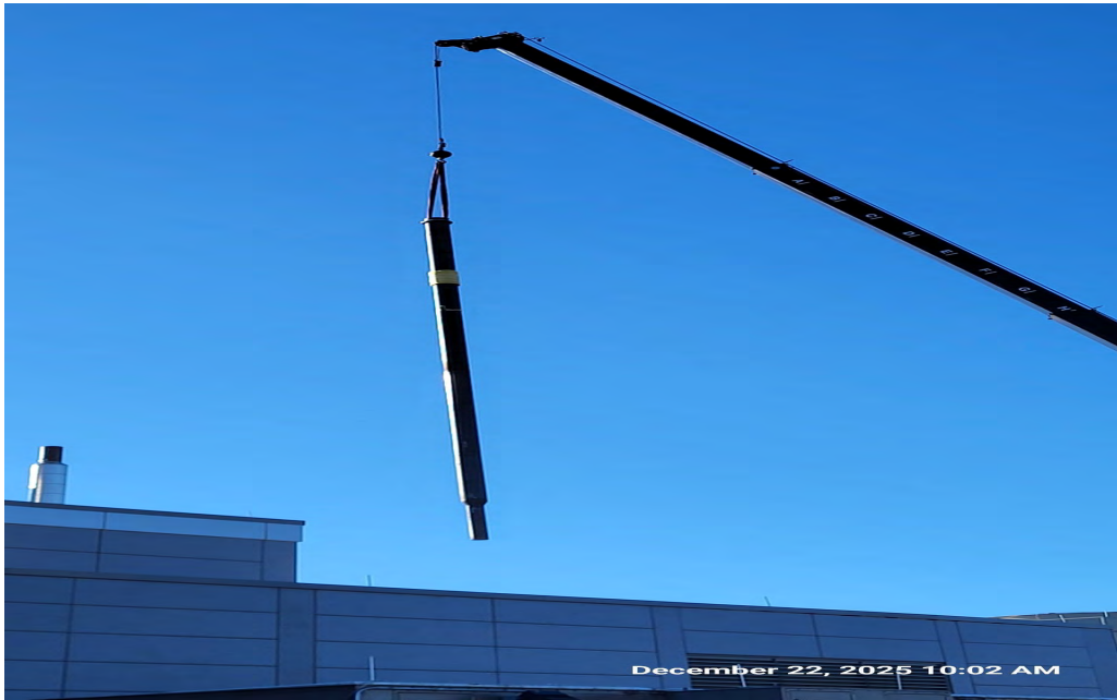
Boiler Relief Bulletin Work @ SUP
