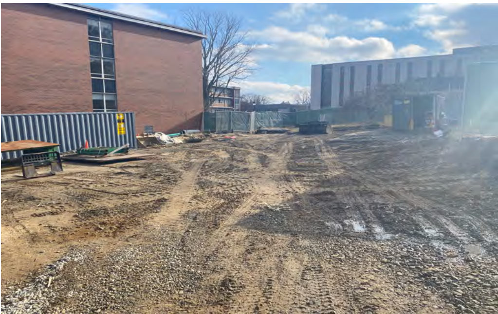
Steam line work completed and backfilled
