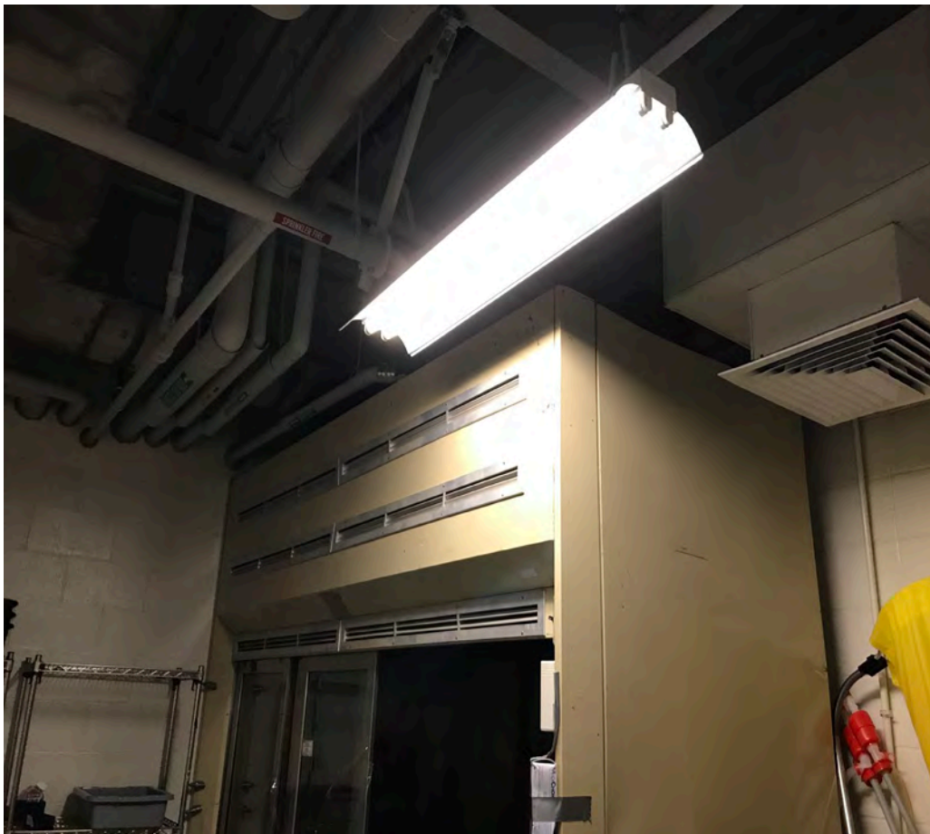
Photo 2 – Existing fume hood to be replaced
