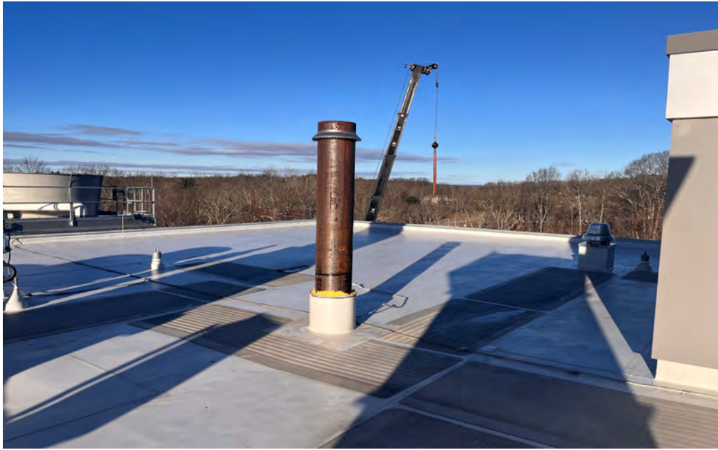
Boiler Relief Bulletin Work @ SUP
