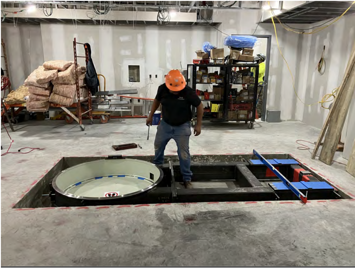
S1868 Vault with LINAC Floor Plate Being Installed
