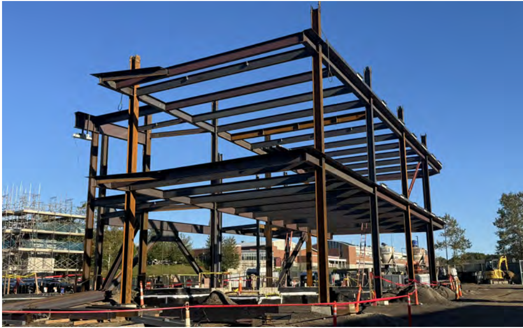
Steel Erection up to Level 2
