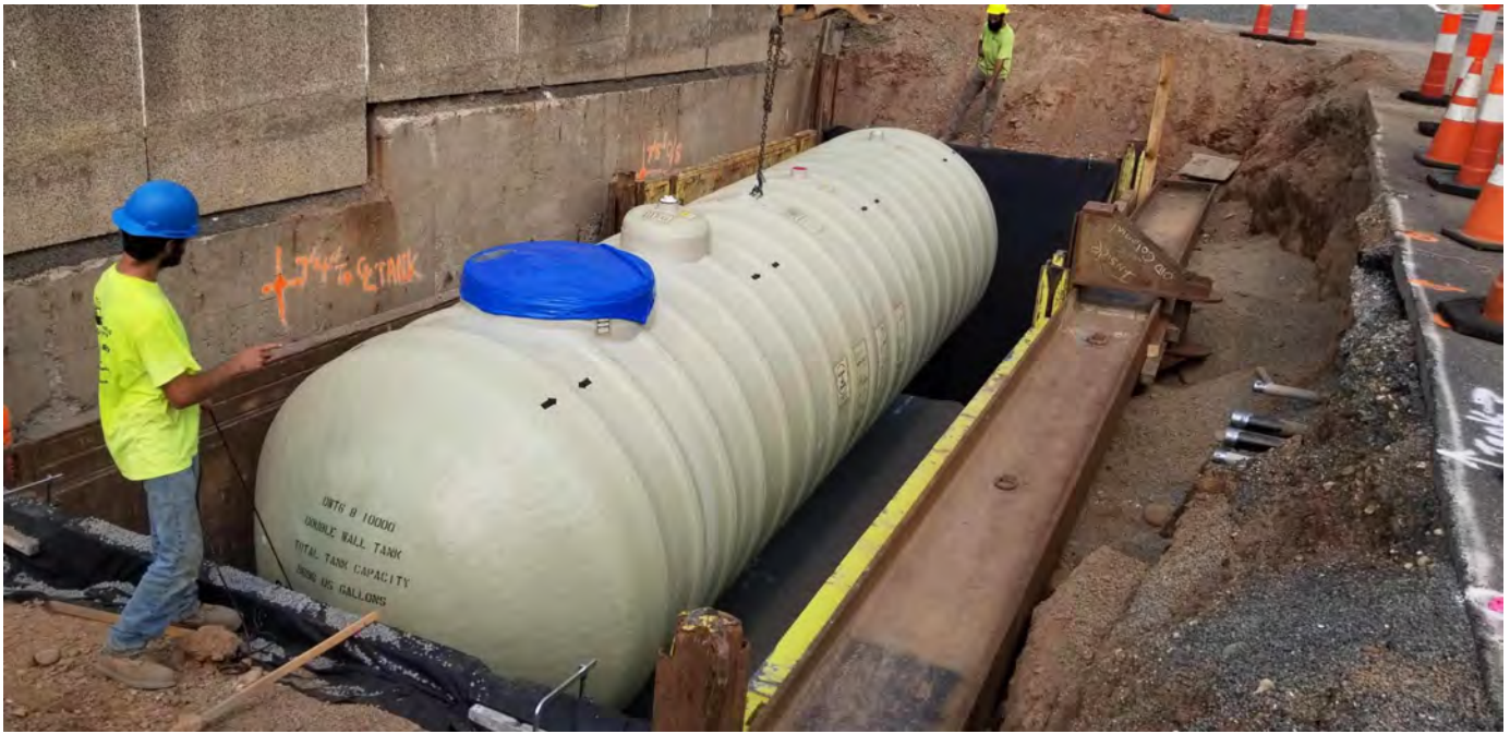
Parking Lot A3 – New UST Installation
