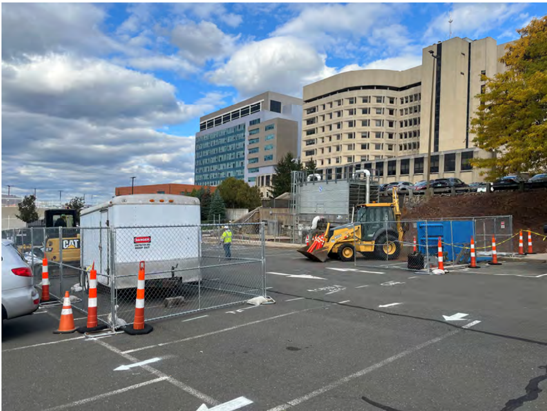
Parking Lot A4 Fenced Construction Area for Oxygen Pad Replacement
