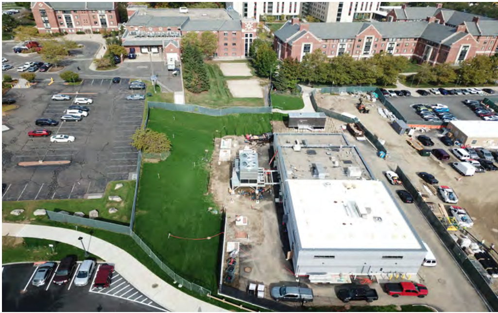
Utility yard is in progress with site finishes installed
