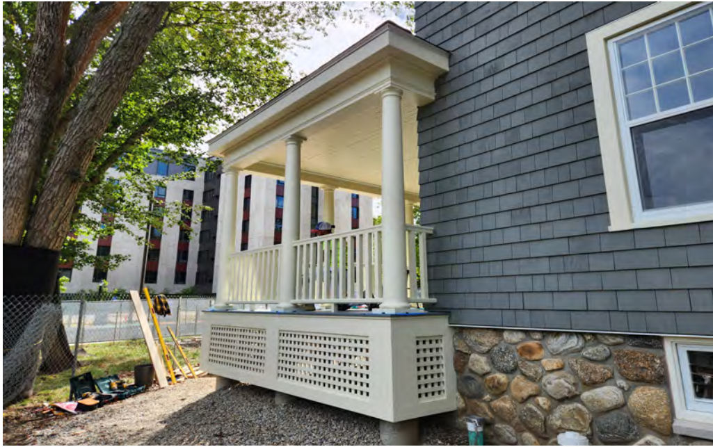
Porches progress - Columns, decking and lattice installation
