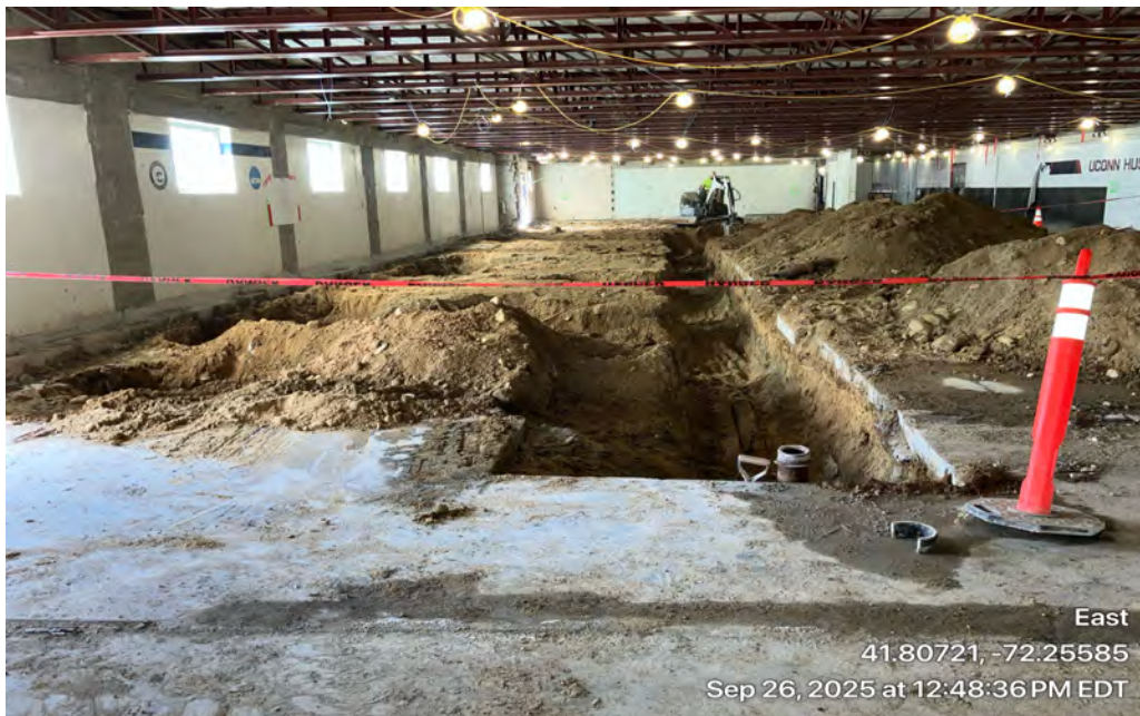
Phase II - Demo & UG Utility Piping Re-Distribution
