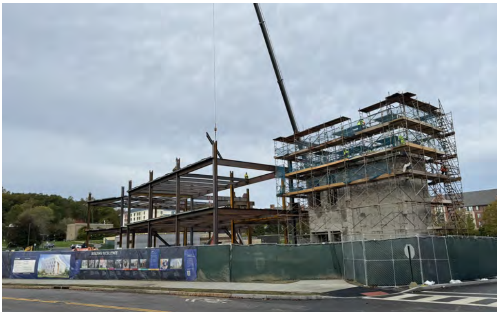
Steel Erection and Masonry Stair Tower (along Bolton Rd)
