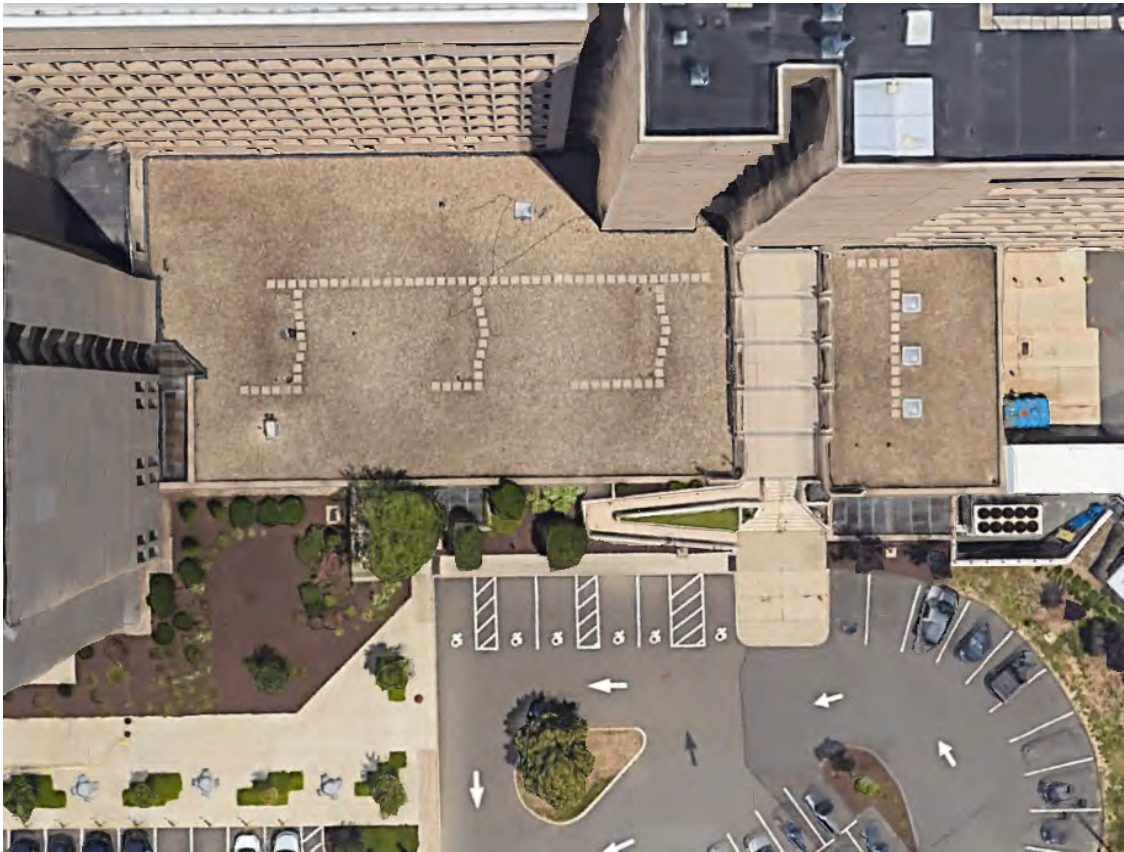
Existing Building K Roof
