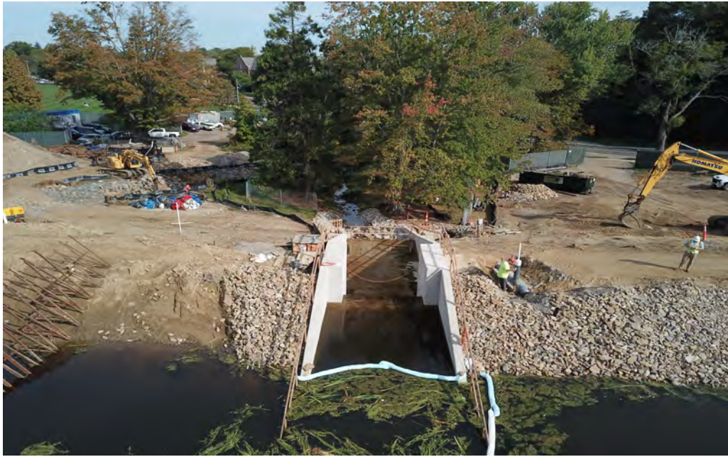
Completed Spillway looking north
