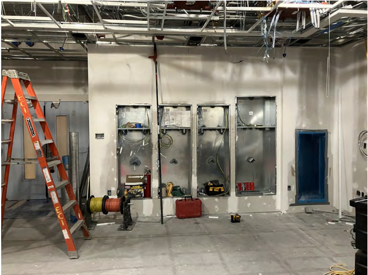
Photo 1 – work in progress showing dedicated electrical panel tubs
