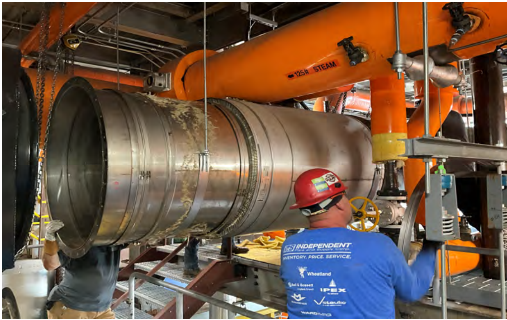
CUP boiler #2 opacity exhaust sleeve replacement
