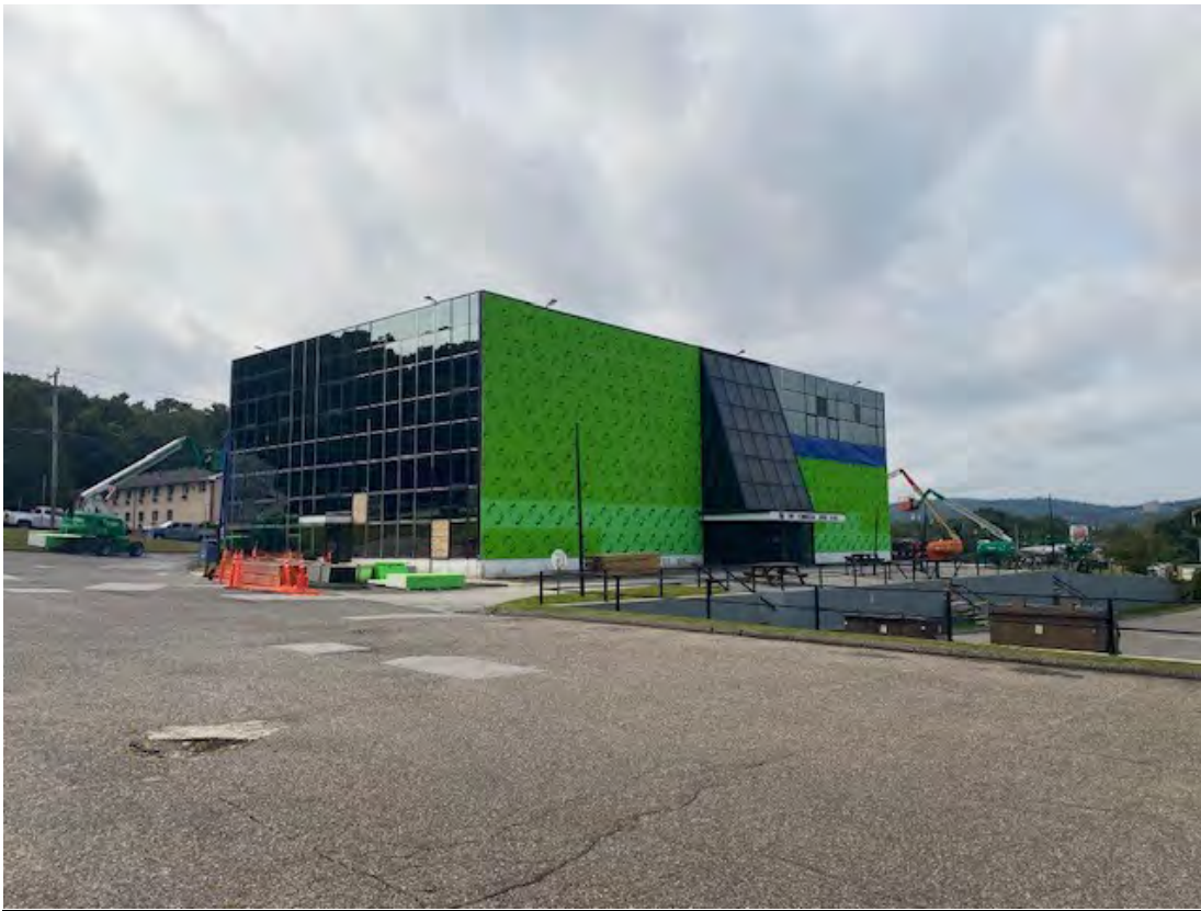
Exterior façade work at front of building
