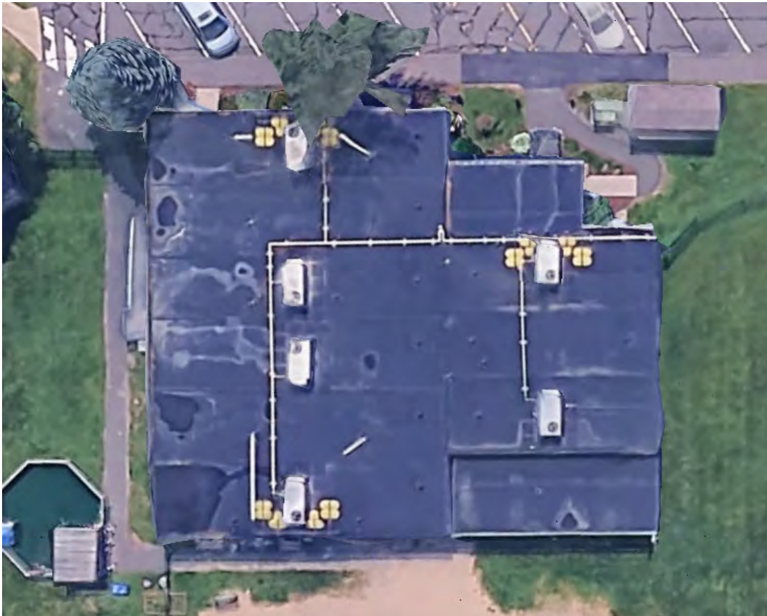
Existing Building M Roof
