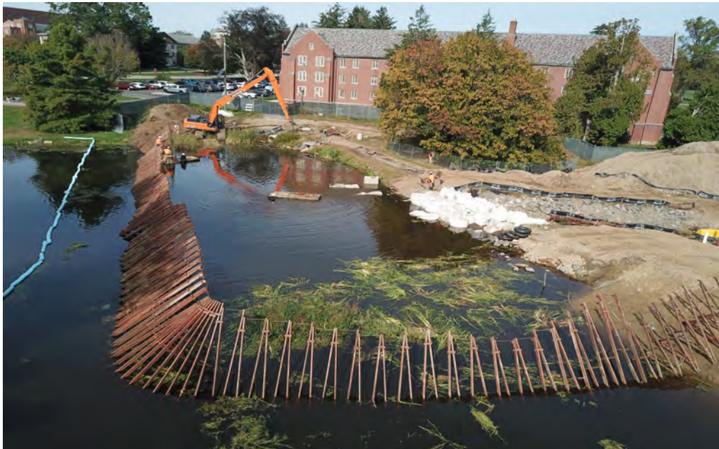
Second Phase of the temporary dam being installed
