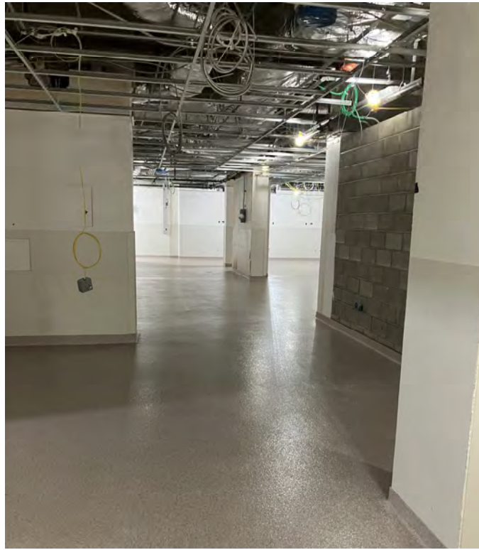
CSS Decon/Clean Newly Installed Epoxy Floor and Ceiling grid
