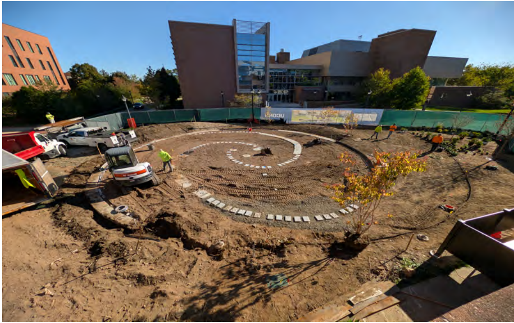
Pavers and Bench Foundation are Complete, Planting has begun
