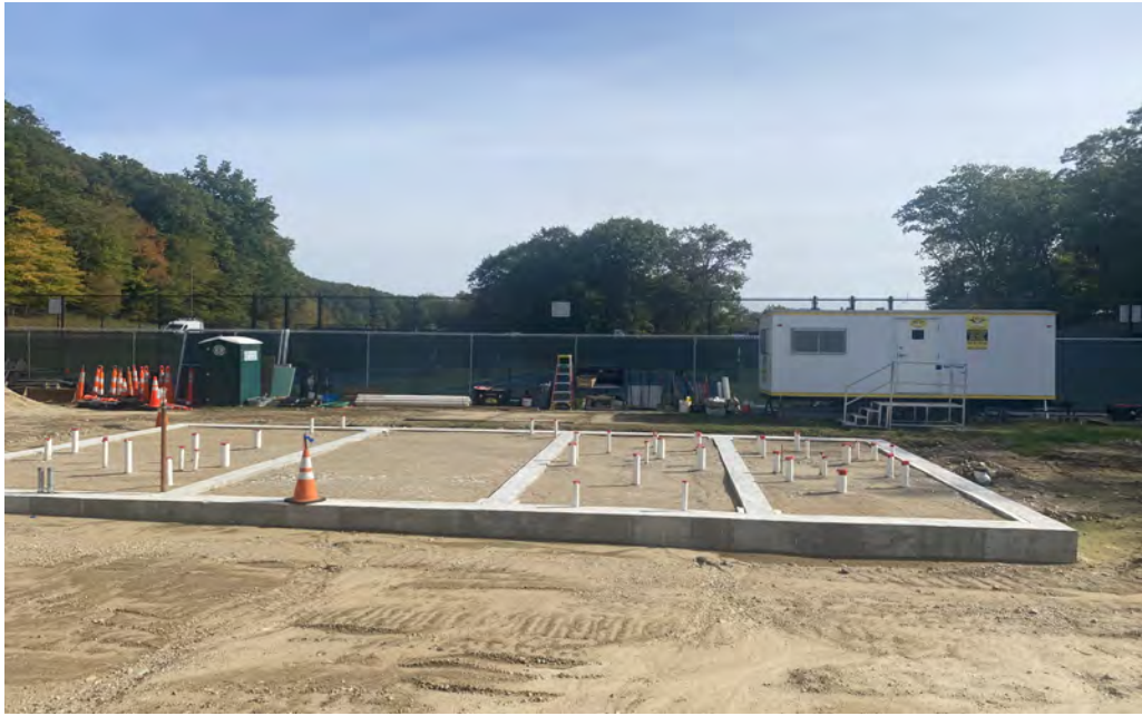
Building underground completed
