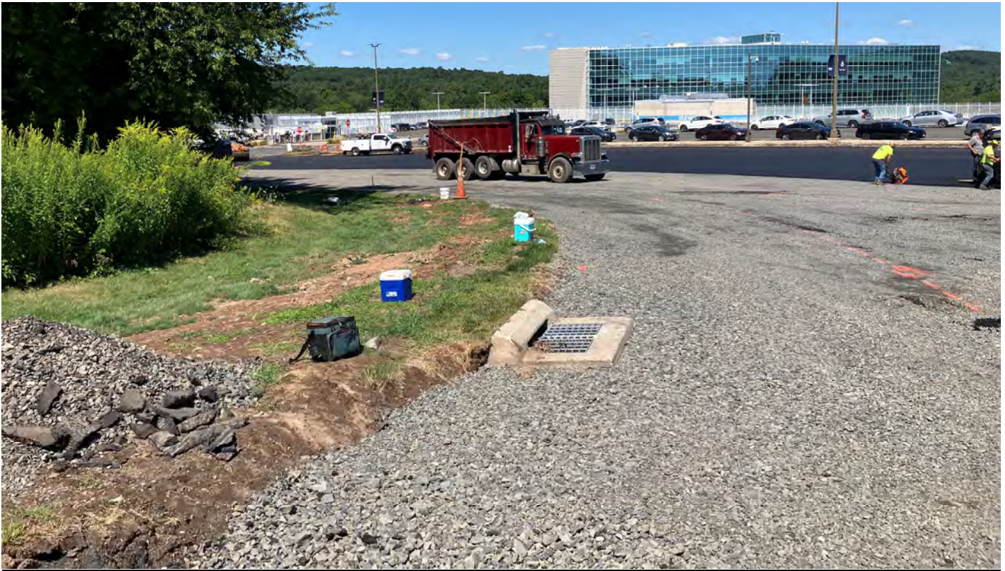
Lot L1 paving binder course.
