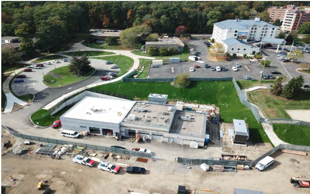
Exterior of building is completed with SON in the foreground
