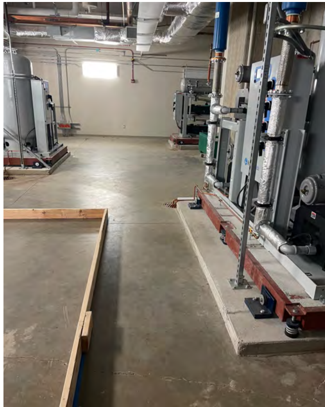
Photo 2 – View of formwork for new CRAC housekeeping pad
