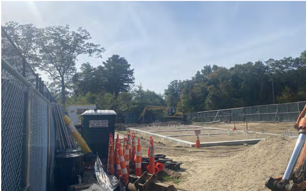
Building underground completed
