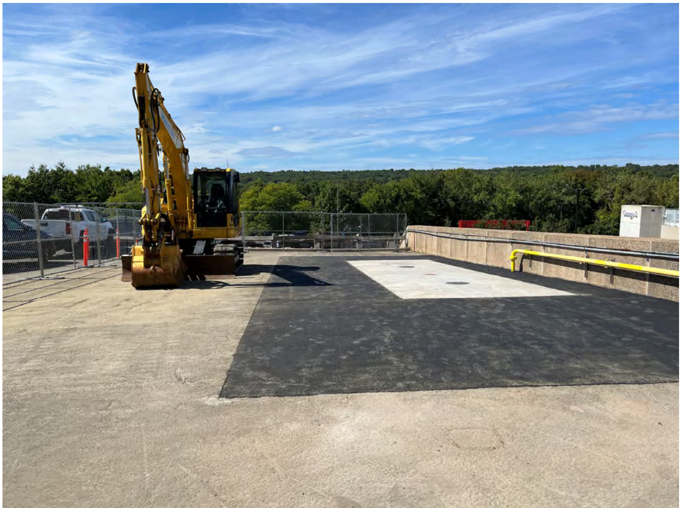
New Concrete Pad and Parking Lot Restoration Above New UST
