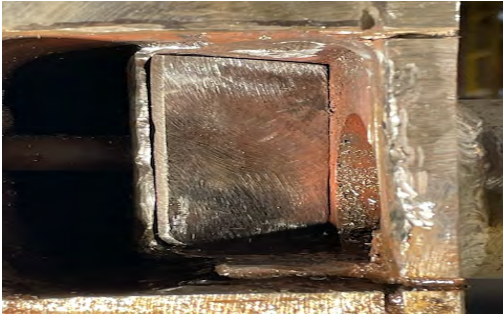
Steel plate to be welded to steam pre-heat coil
