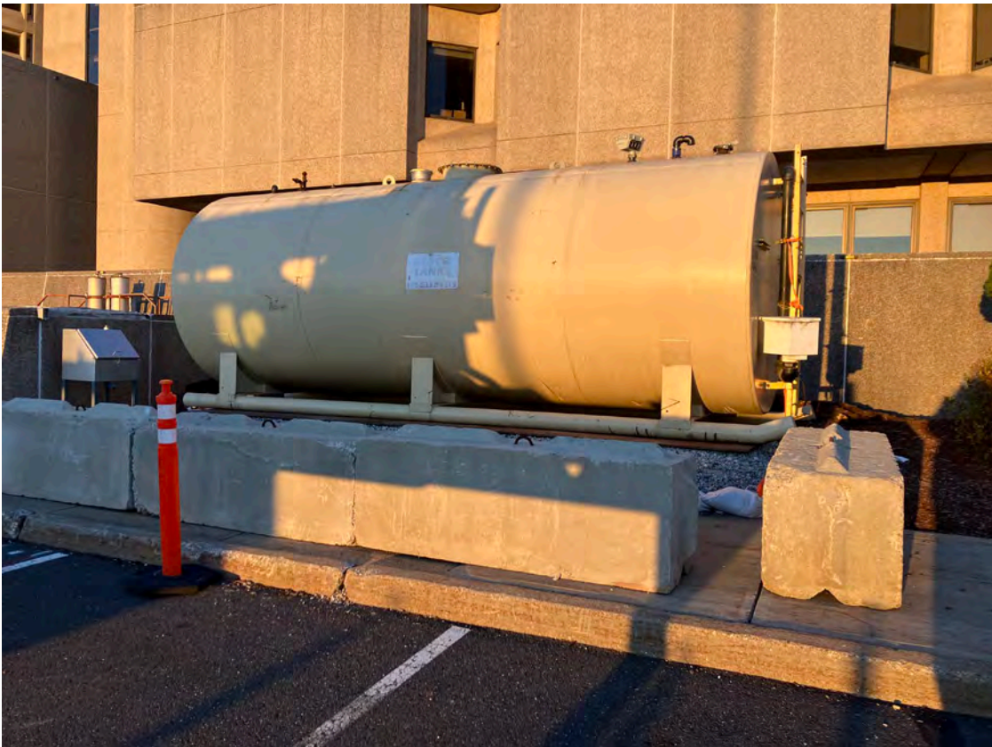
Temporary Above Ground Fuel Storage Tank Placed for Hookup
