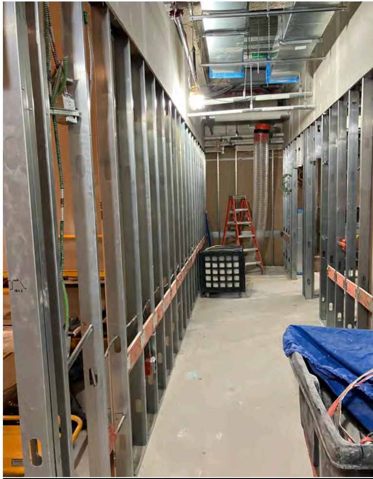
New corridor with exam rooms on either side framed and utilities roughed in walls
