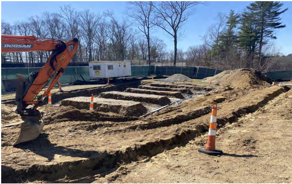
Foundation excavation prepared for forms and concrete.
