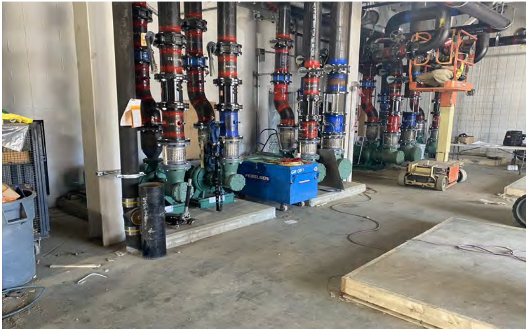
Chilled and Hot water pumps installed
