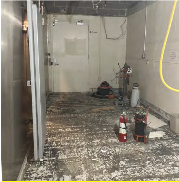
Phase 2 – Tile Floor Removed in Morque Room CG048
