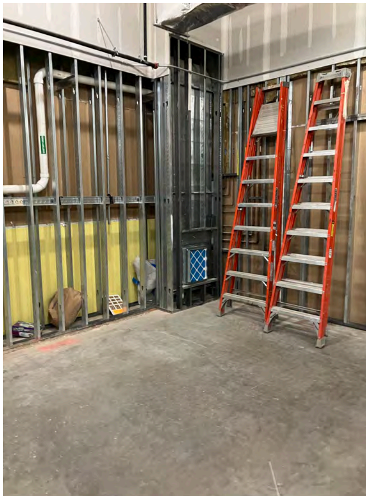
Photo 2 – Interior demising wall at exhaust duct.
