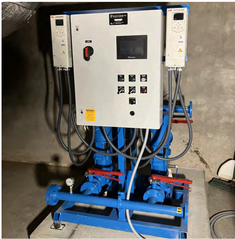
New Booster Pump Serving Endoscopy Scope Sterilizers
