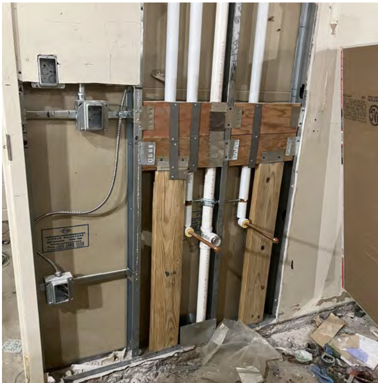
Phase 2 - New Plumbing for Hand Wash Sink in Autopsy CG047
