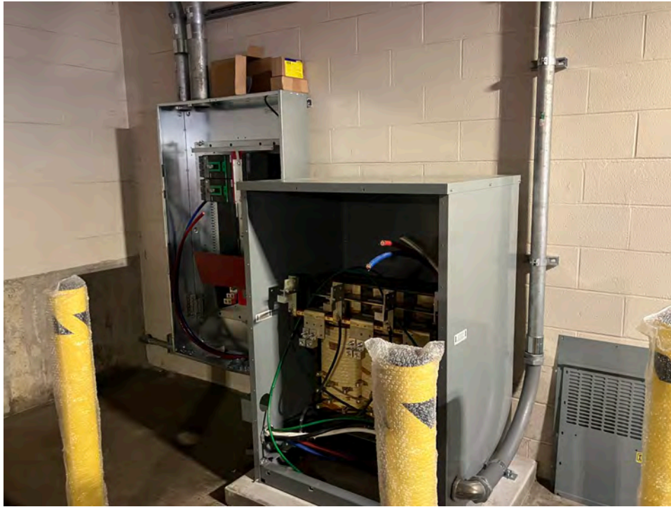
Garage 1 New transformer and panel
