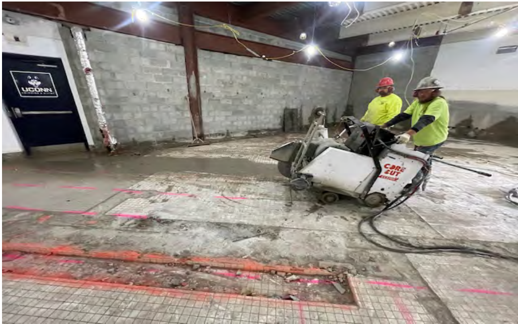
Swim Locker area slab cuts for continued demo.
