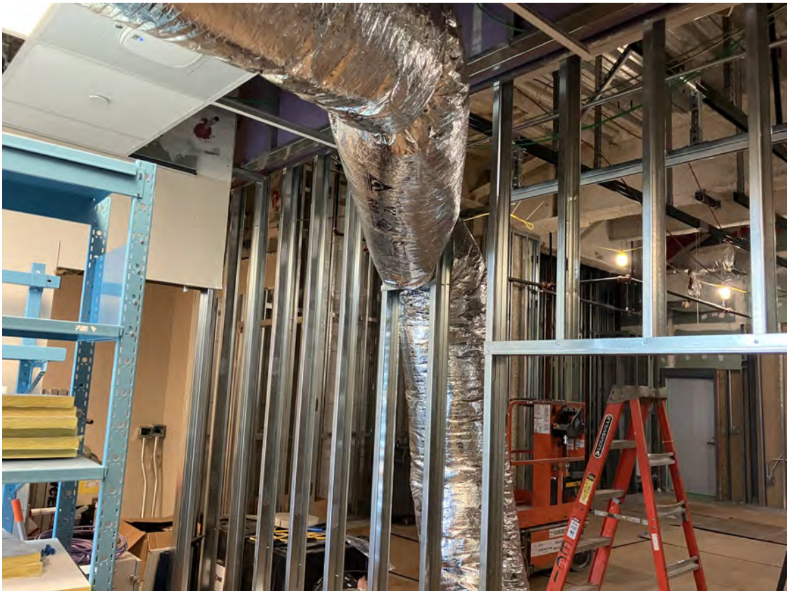
Photo 2 – Interior demising wall framing at Clinical Engineering demising wall.
