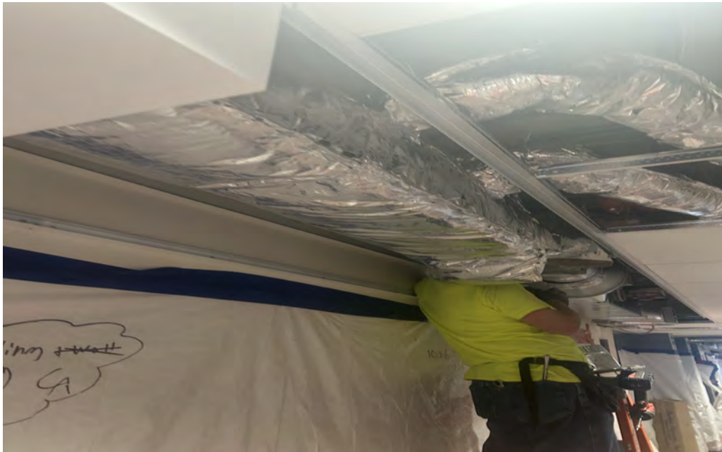
New Ducts That Will Bring Fresh Air to Student Rooms
