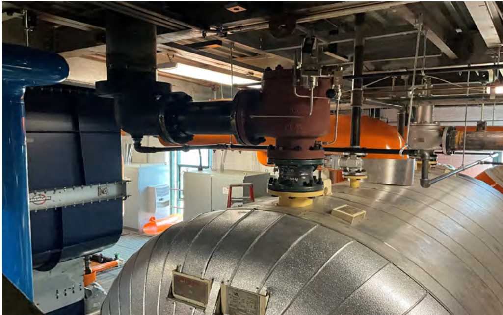
Relief valve installed at CUP deaerator tank.
