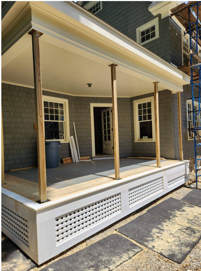
Porches progress - decking and lattice installation
