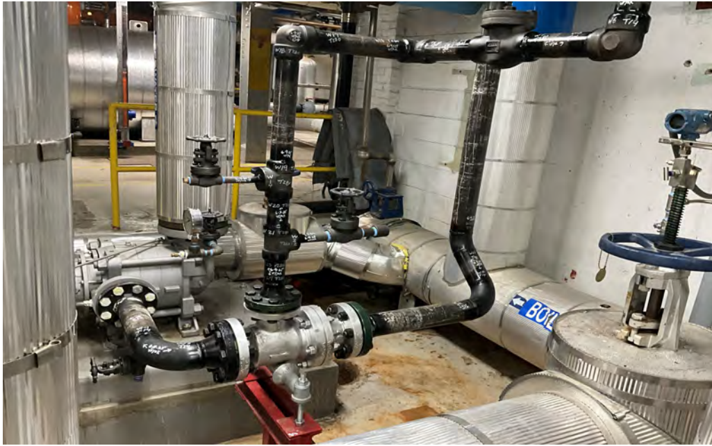
ARC valve and piping installation at CUP feedwater pump.
