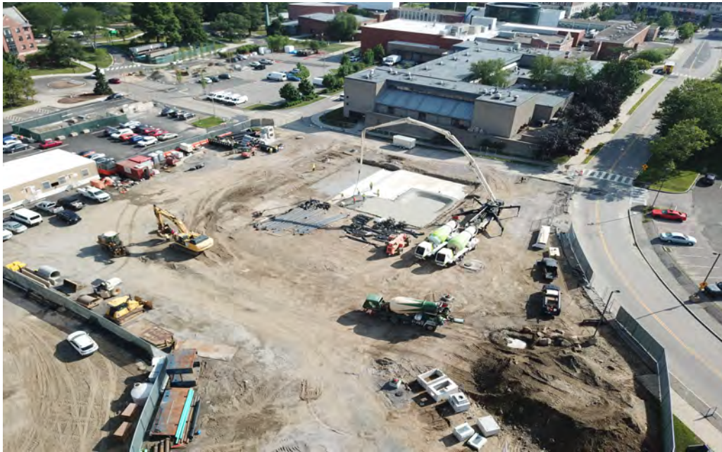
Drone Photo 7/8/25 - Pouring of concrete mat slab
