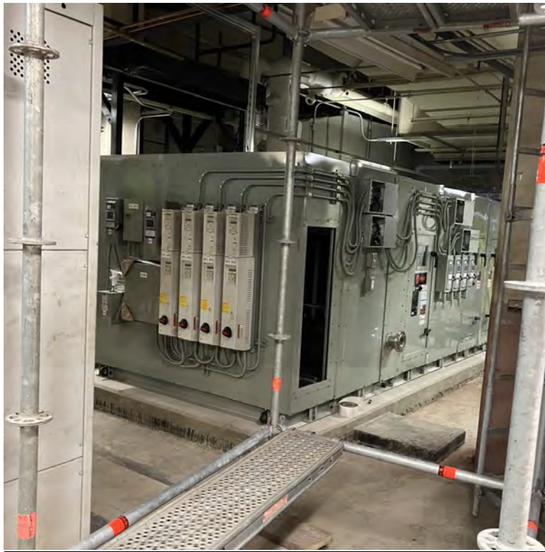
Phase 2 New Blower 57 set on Equipment Pad in C-Basement
