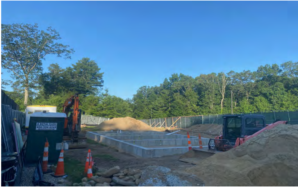
Foundation complete and under slab plumbing has started
