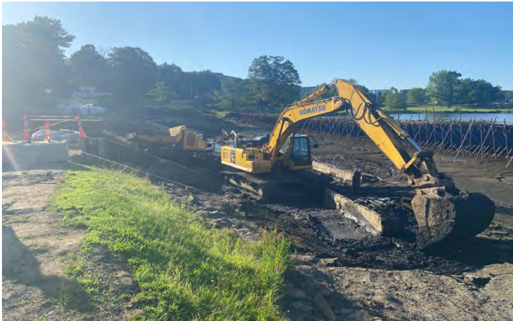
Sediment being removed in dam work area
