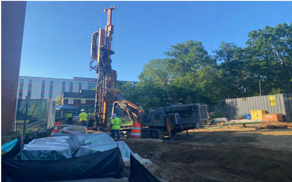
Support of Excavation being installed
