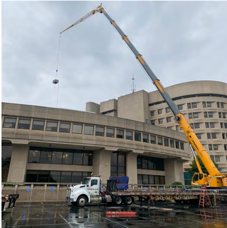
Phase 2 Crane Pick in Lot M2 for New AHU and Demolition
