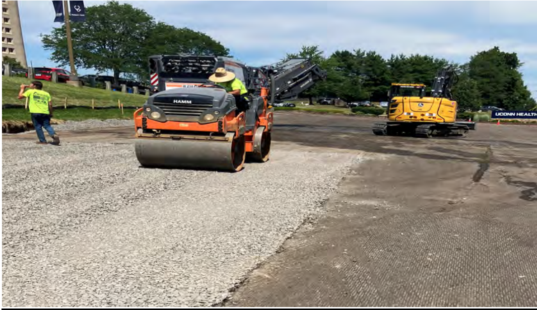
Lot A5 after milling and a soft spot of base being replaced.
