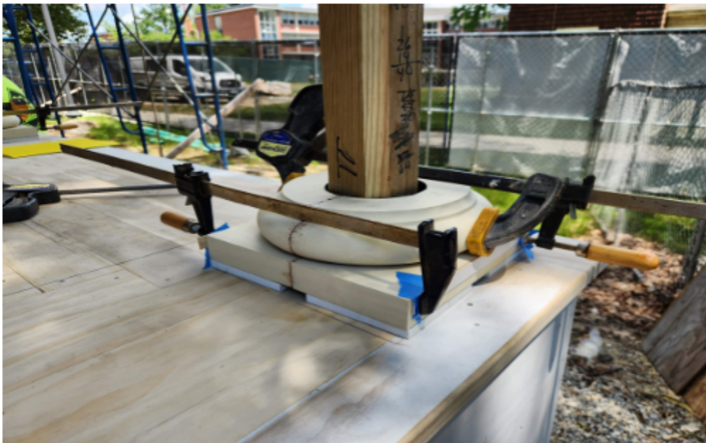
Column base installation mock- up
