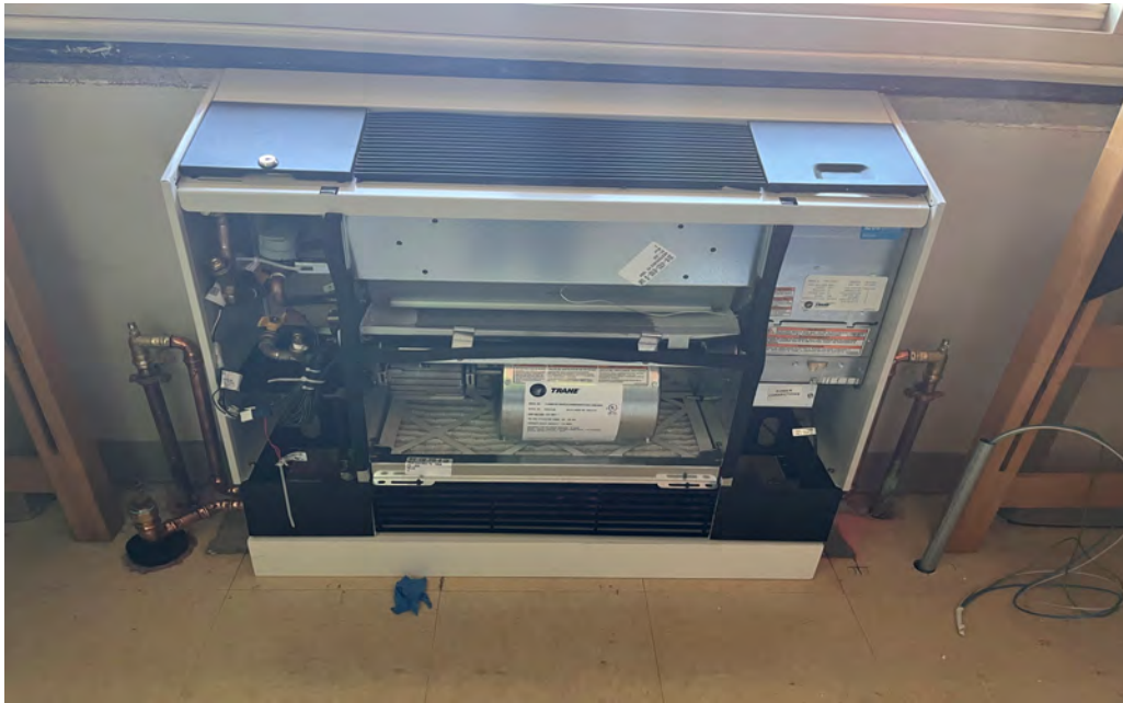
Typical Dorm Room Fan Coil Unit
