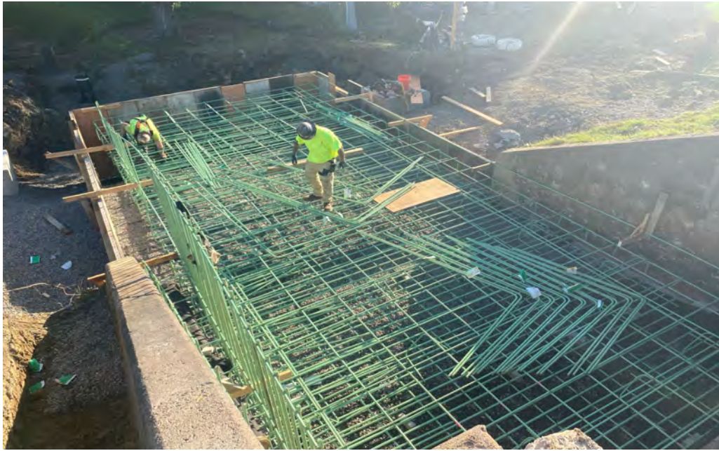
Downstream rebar being installed
