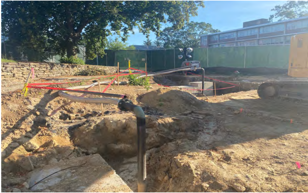
Temporary Steam Bypass installed and operational
