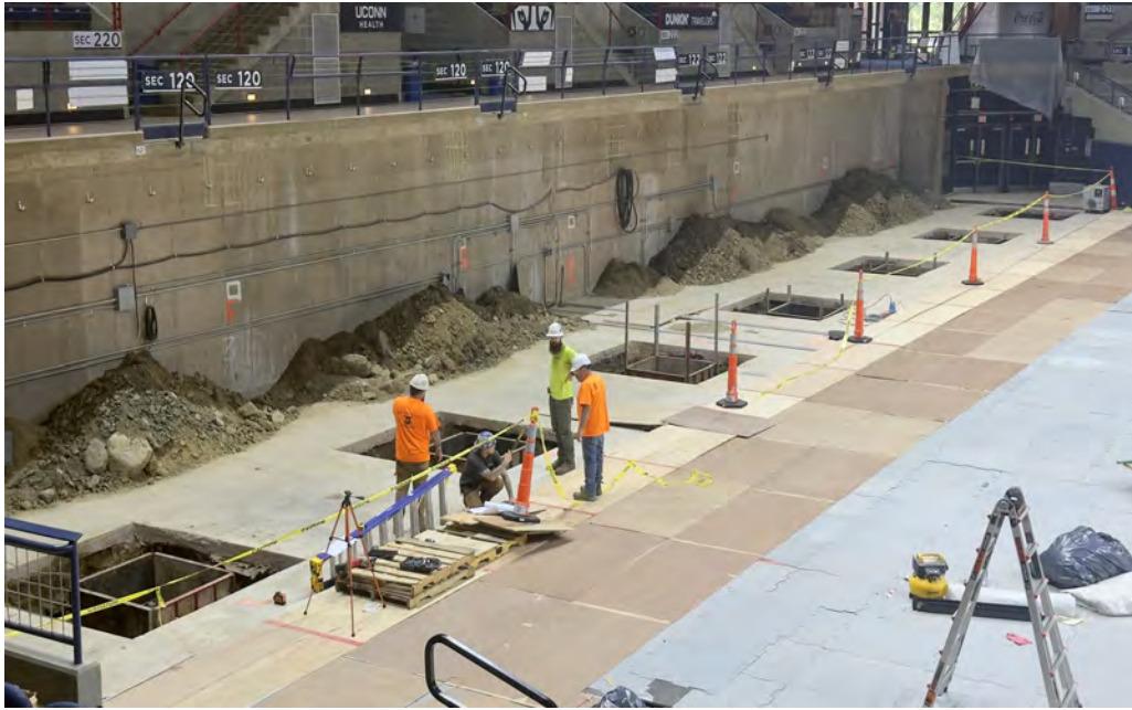
Footing Locations for Steel Beams on North Side
