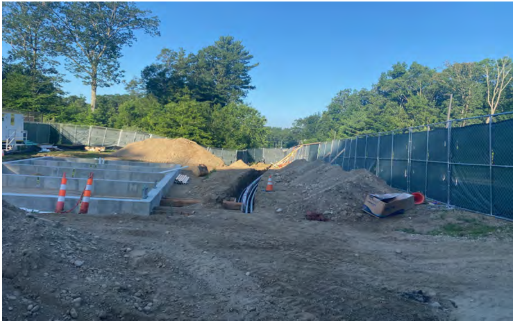
Power and Telecom duct banks installed
