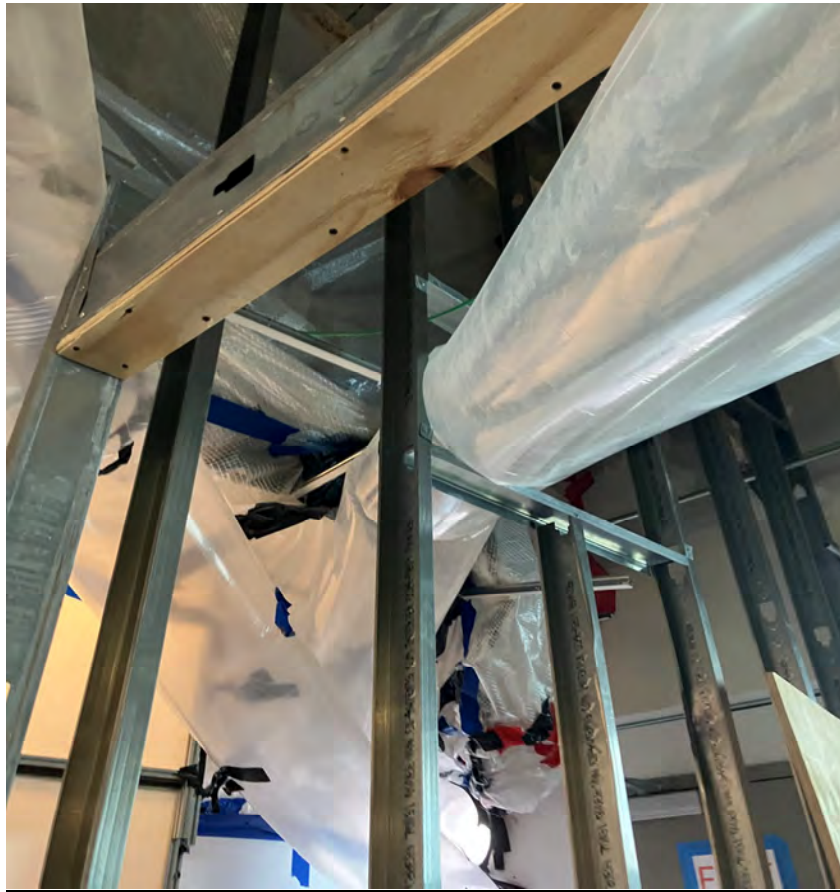
New Steel Stud Framing with Negative Air Exhaust Shown
