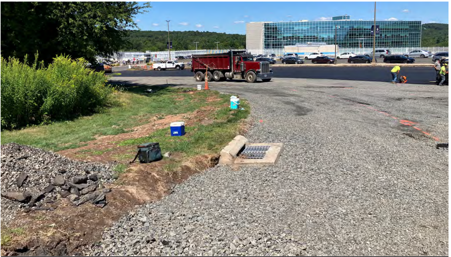
Lot L1 paving binder course.
