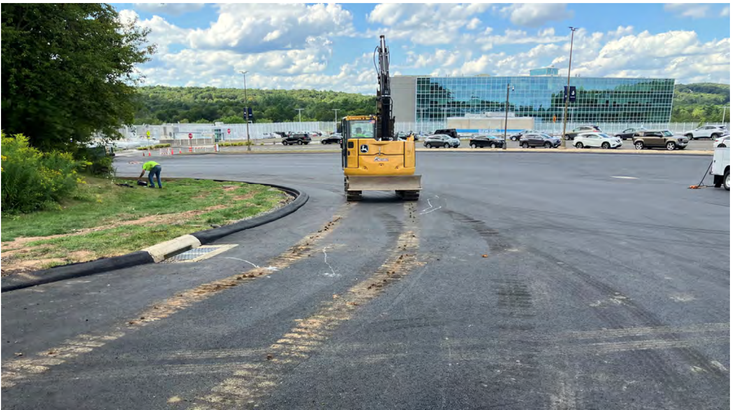
Lot L1 paved and curbing installed. Topsoil and lawn restoration.
