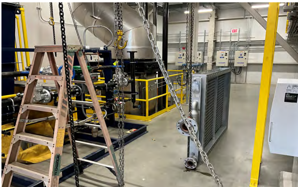
SUP faulty steam coil replacement
