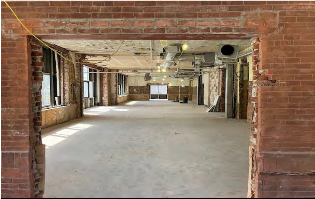
Interior first floor space – view of future radiology area.
