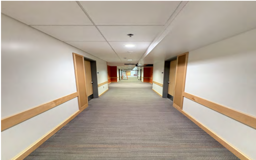
New duct with metal soffit
