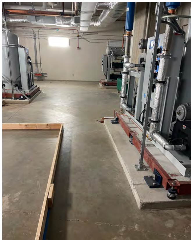
Photo 2 – View of formwork for new CRAC housekeeping pad
