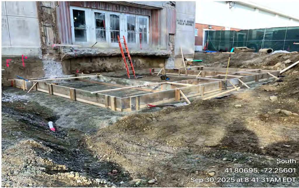
Phase II - Main Entry Footing Form Work
