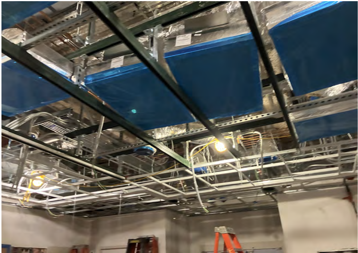
Photo 2 – New laminar flow HVAC system rough-in
