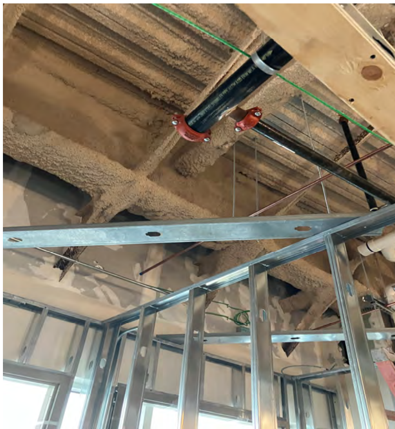
New Steel Stud Framing Showing Bracing & Borrowed Lights
