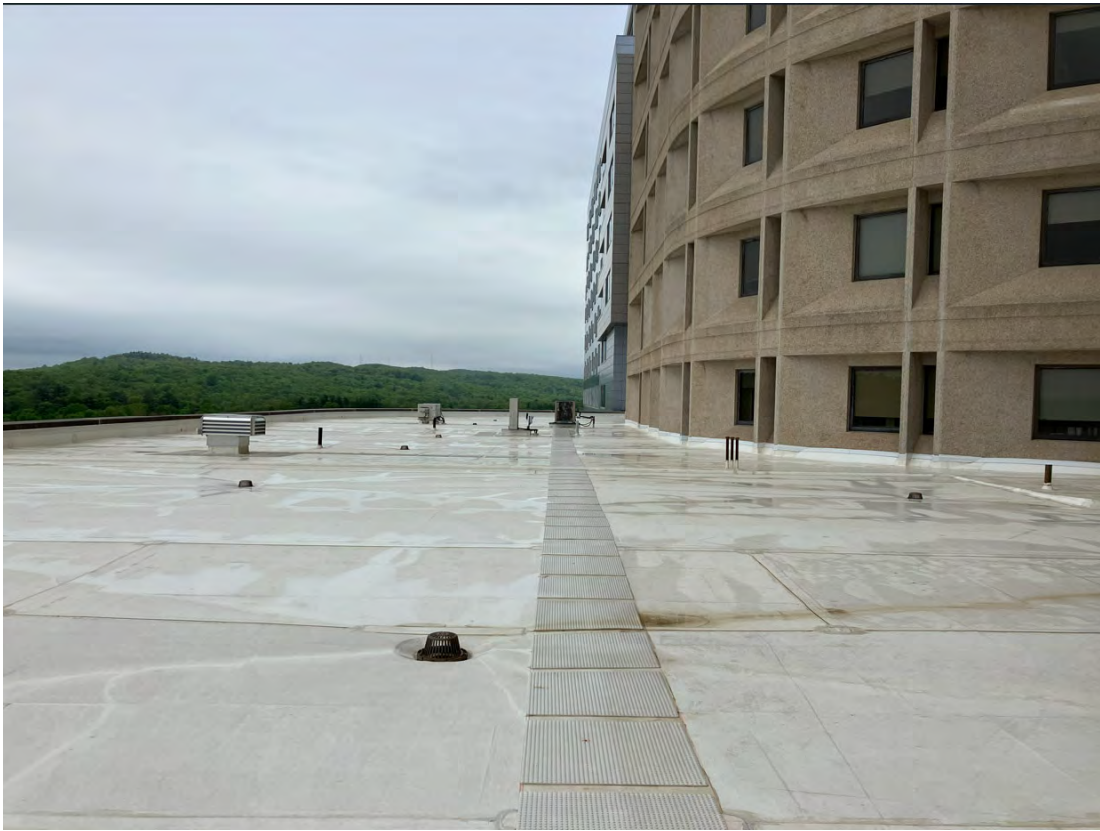
Completed Building F Roof
