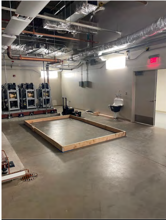
Photo 1 – View of formwork for new CRAC housekeeping pad
