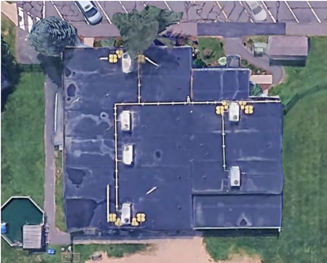
Existing Building M Roof
