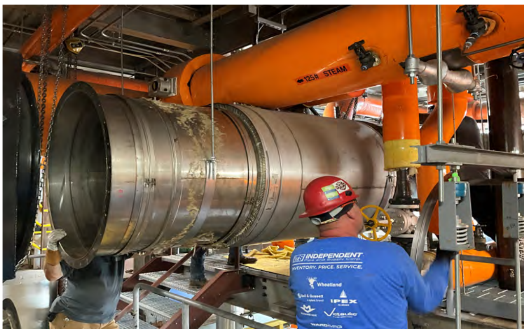
CUP boiler #2 opacity exhaust sleeve replacement
