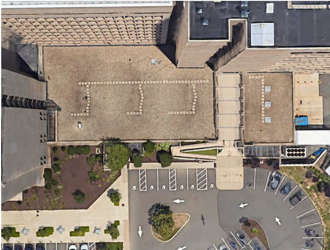
Existing Building K Roof
