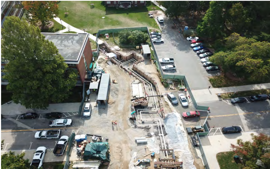
Vault E8 with steam pipe to the north
