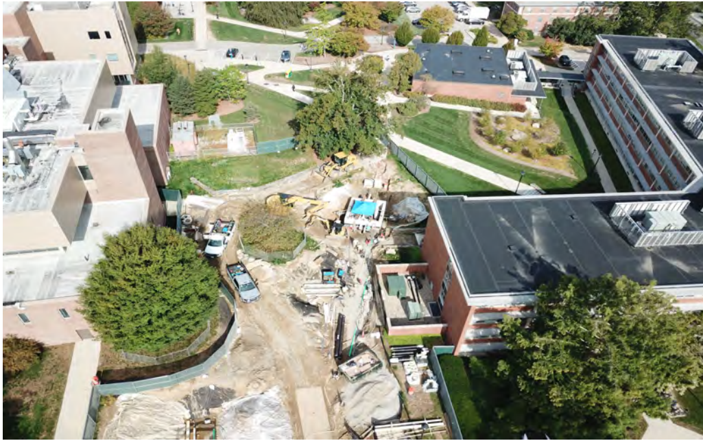
Vault Q8 progress with final steam connections to existing
