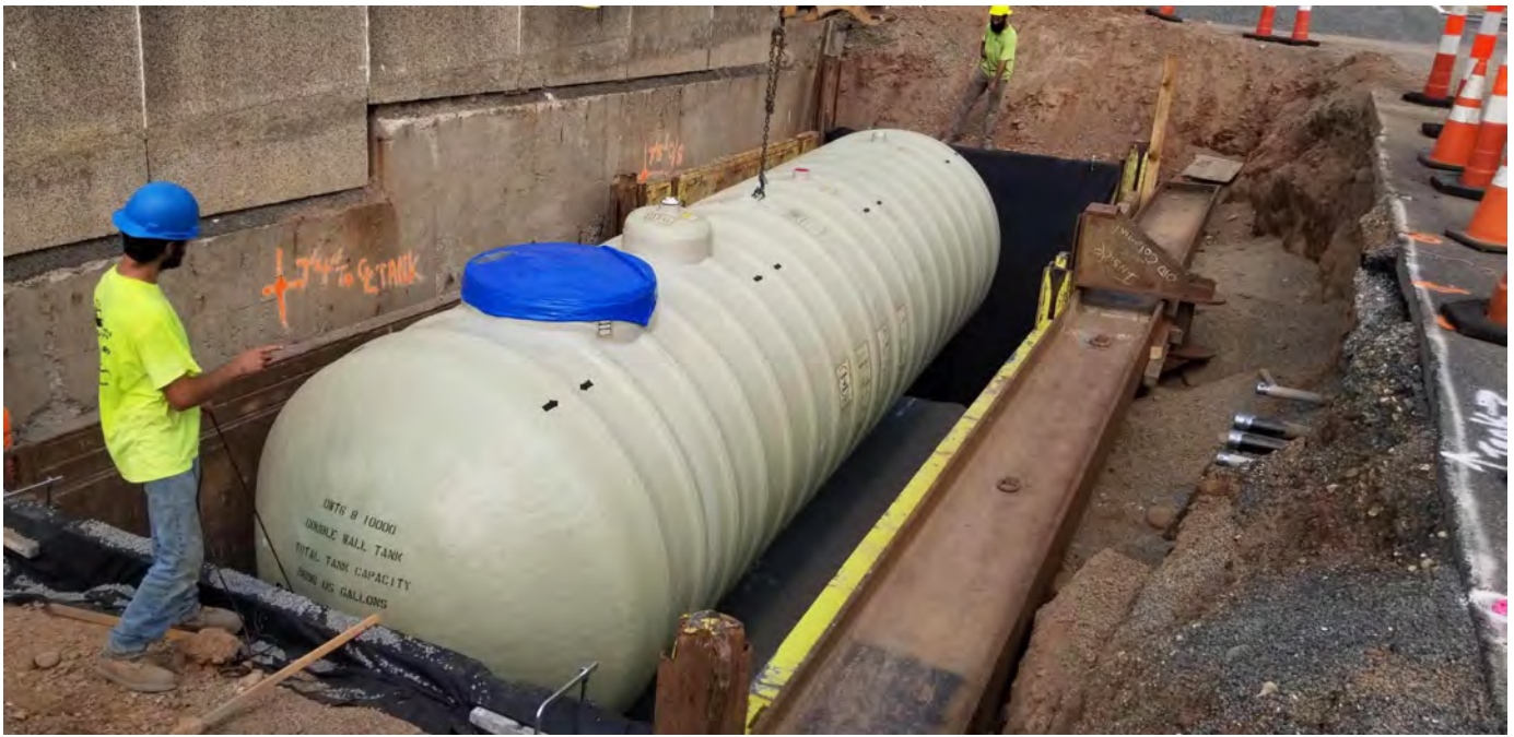
Parking Lot A3 – New UST Installation
