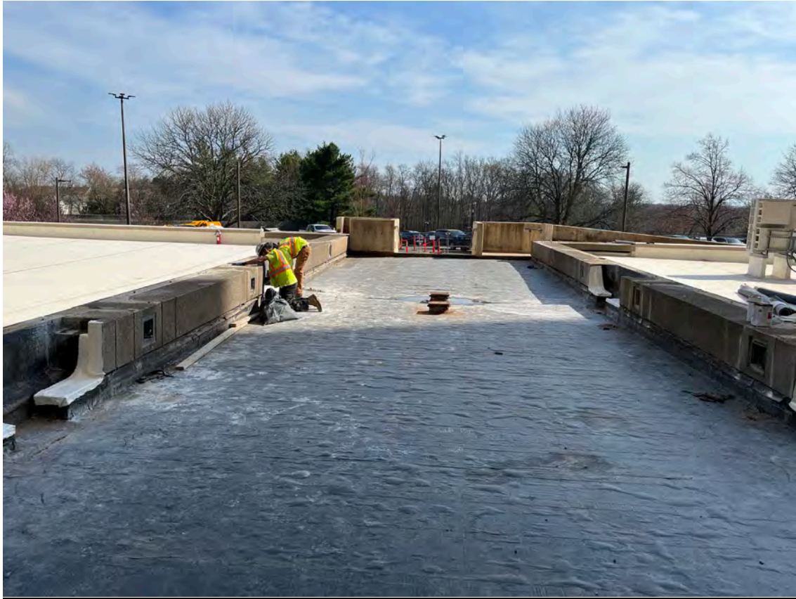
Entrance Walkway Removed, Curb Removal in Progress
