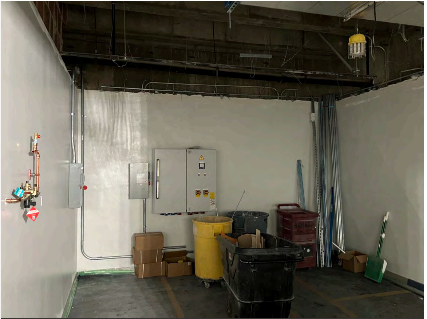
BB013 MRI Room Progress
