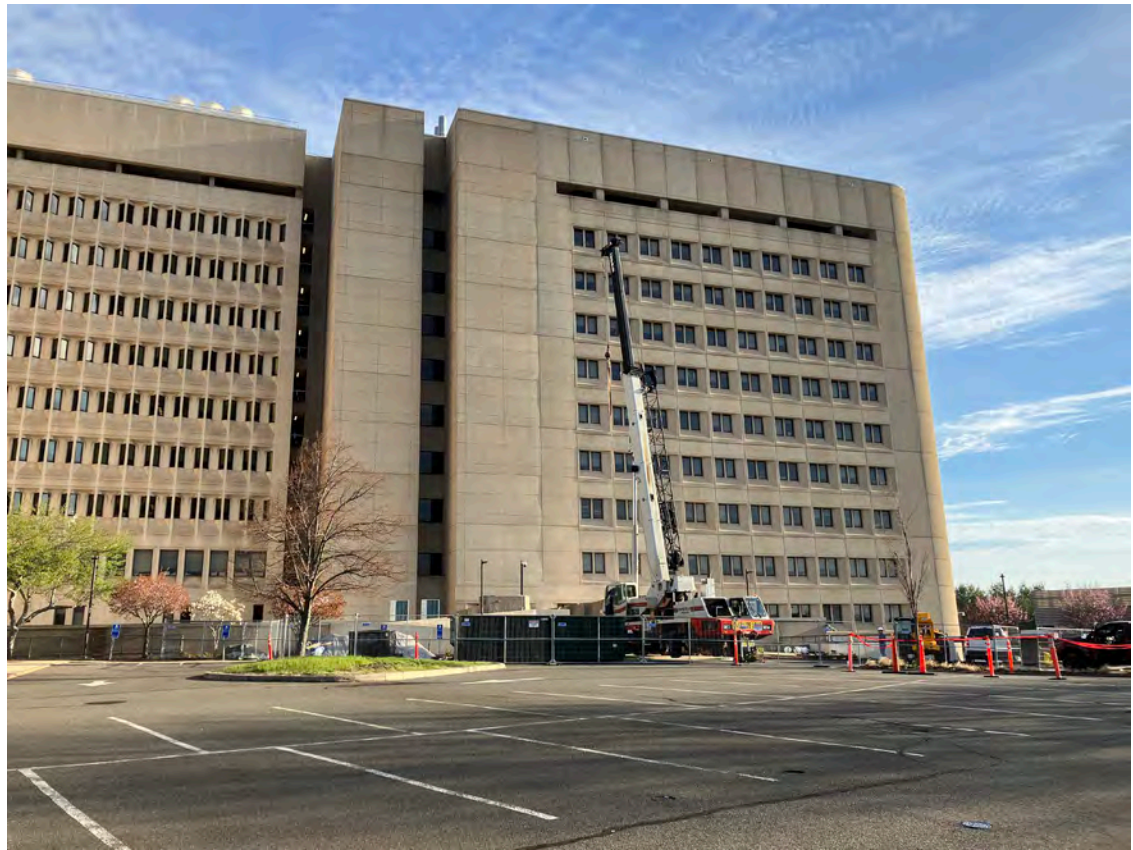
Building E & Building K Construction Area in Parking Lot A2
