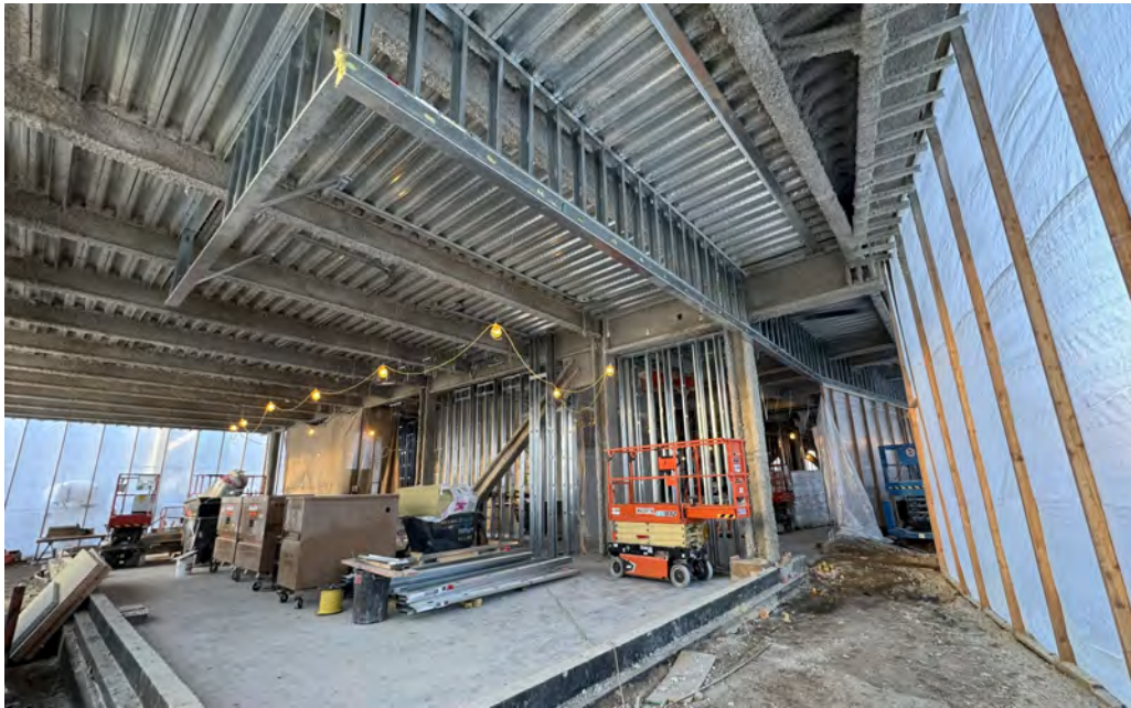
Interior metal framing/fireproofing on steel above- Level 1
