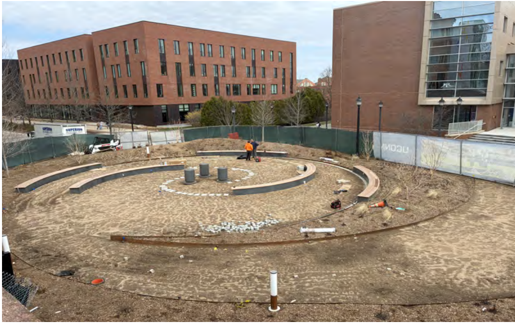
Electricians installing the bench lights
