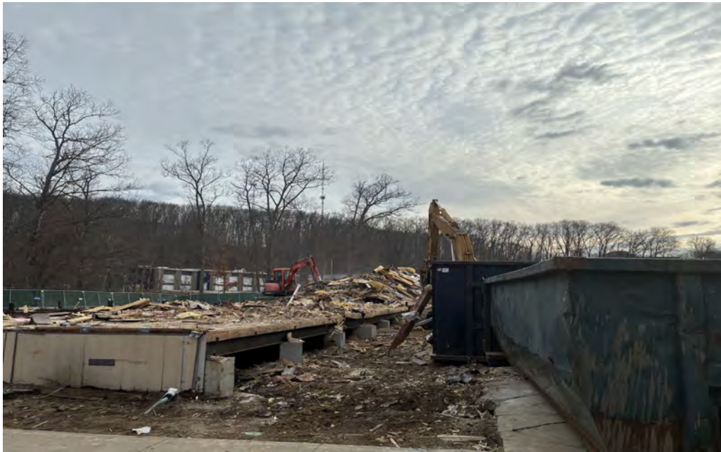
Second Week of Building Demolition
