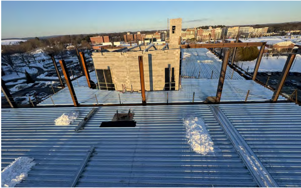
Steel framing & metal decking - Looking East
