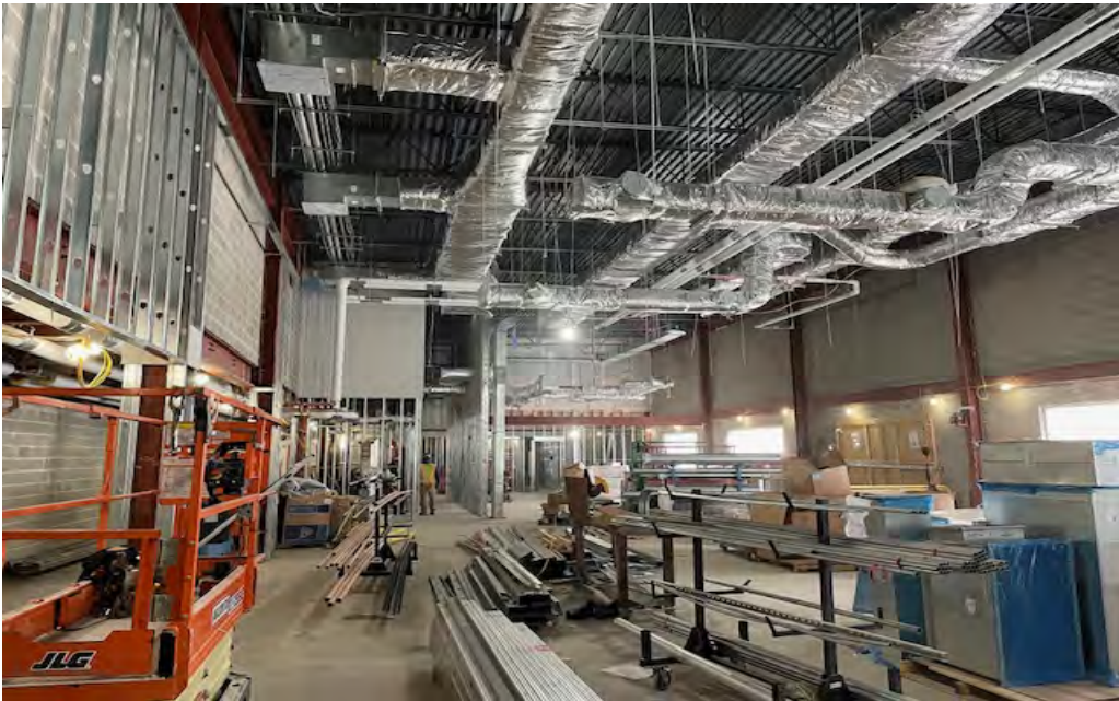
Phase II - Open Academic Study Area Ductwork in Progress
