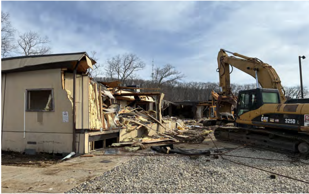
First Week of Building Demolition
