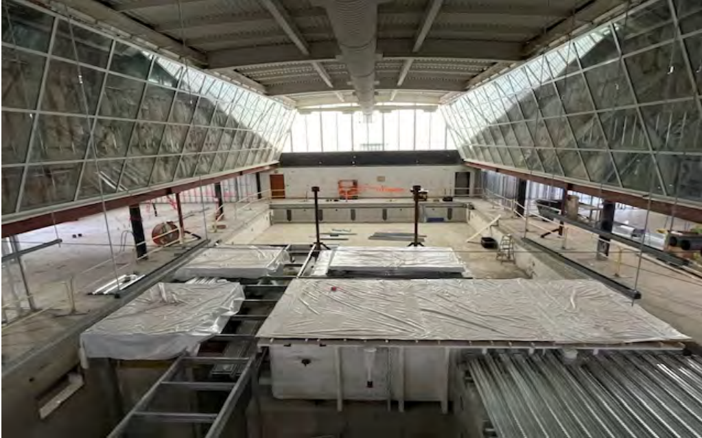
Phase II - Hydrotherapy Tanks In Place & Protected
