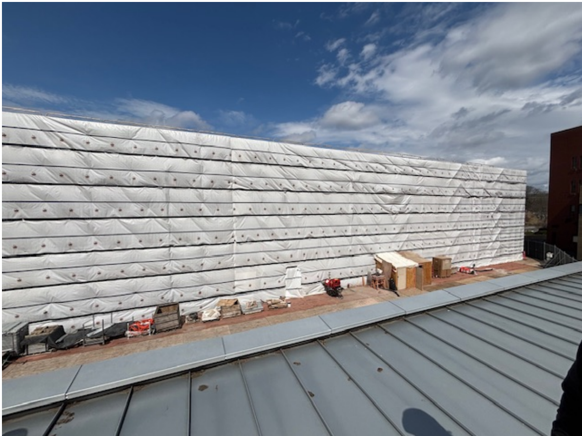
Gant North Exterior Scaffolding & Thermal Plastic Envelope Wrap
