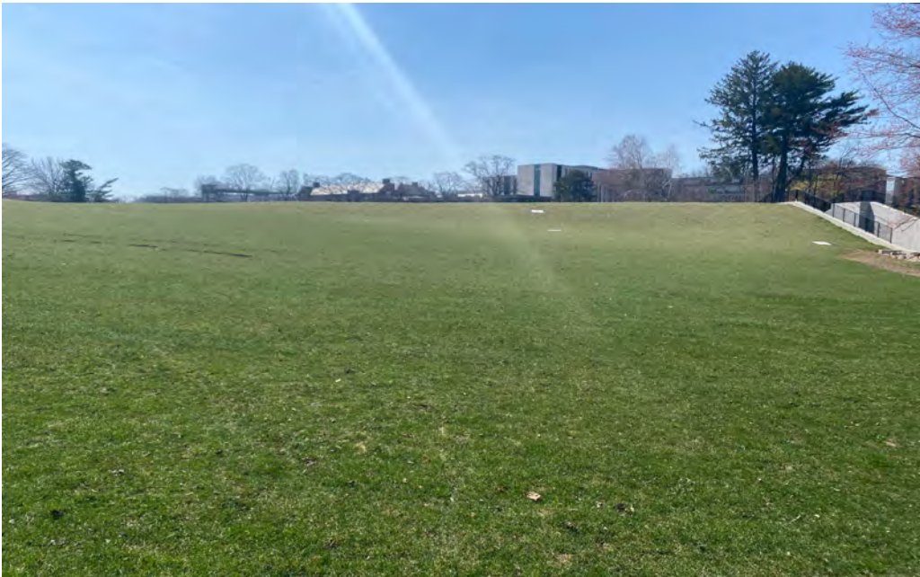
Eastside of spillway
