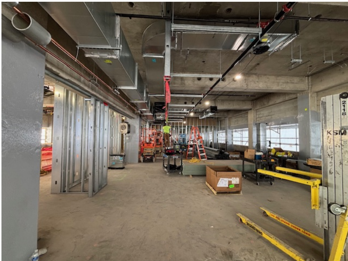
Gant North 2nd Floor Framing & Duct Installations
