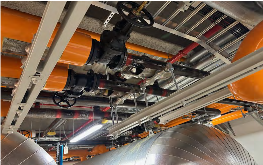
Valve Replacement Work @ SUP per Bulletin
