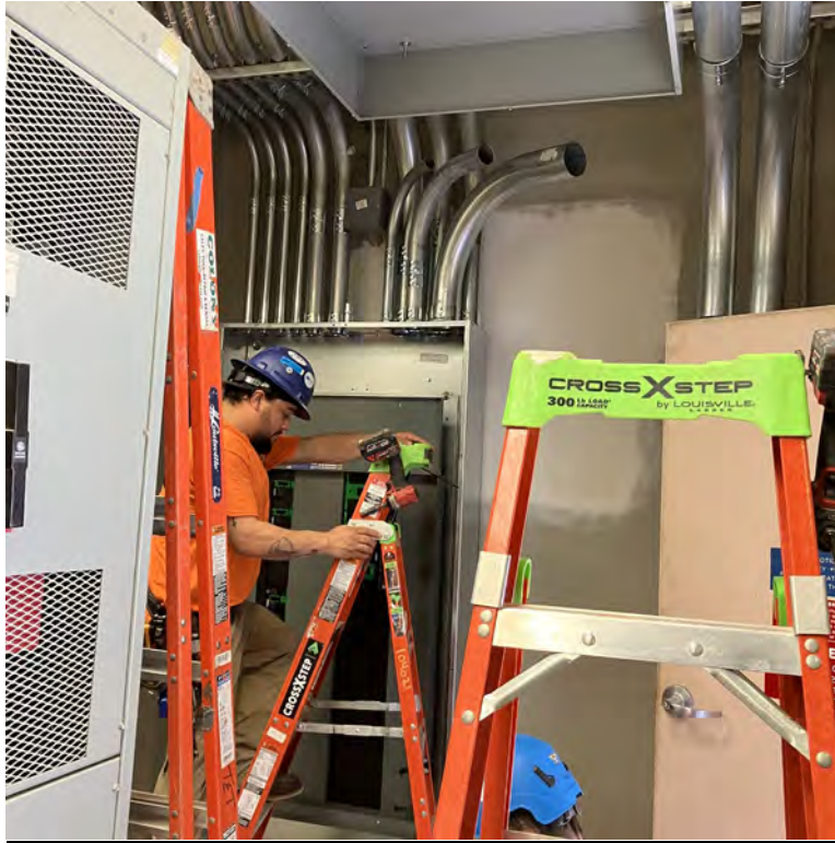
Installation of new ATS in Main Switch Gear Room
