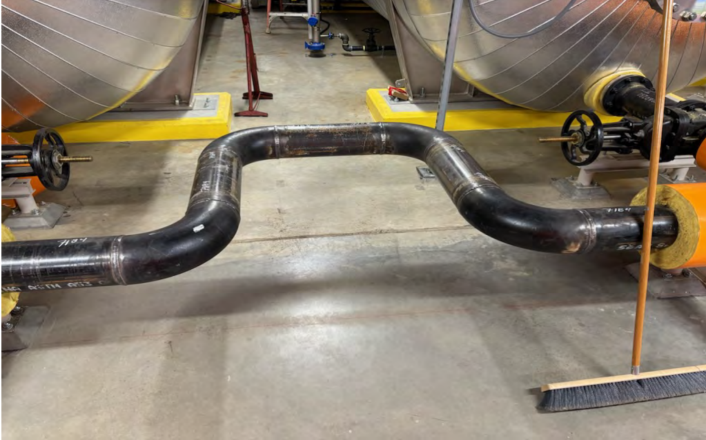
Stress Analysis Loop being added @ SUP
