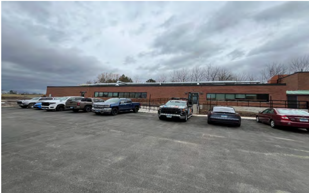
Front of Building
