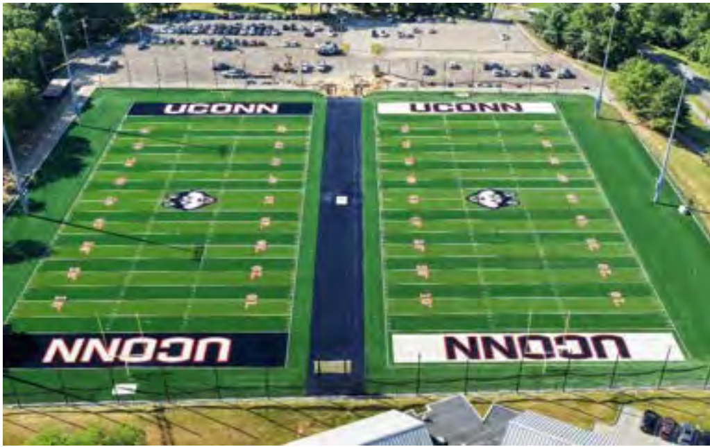
Turf complete,. entry way upgrades in progress
