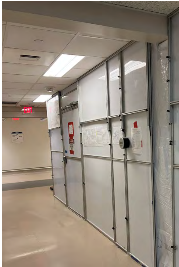
Temporary Construction Barrier at Future Reception Area
