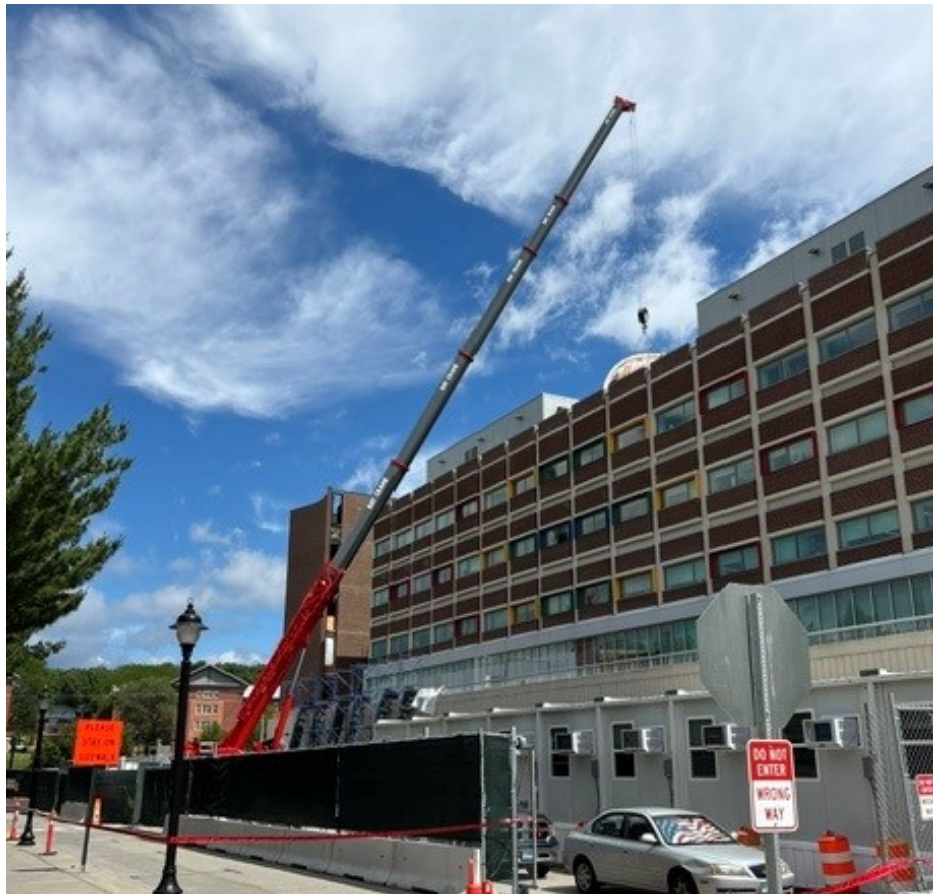
Gant West Observatory Dome Removal
