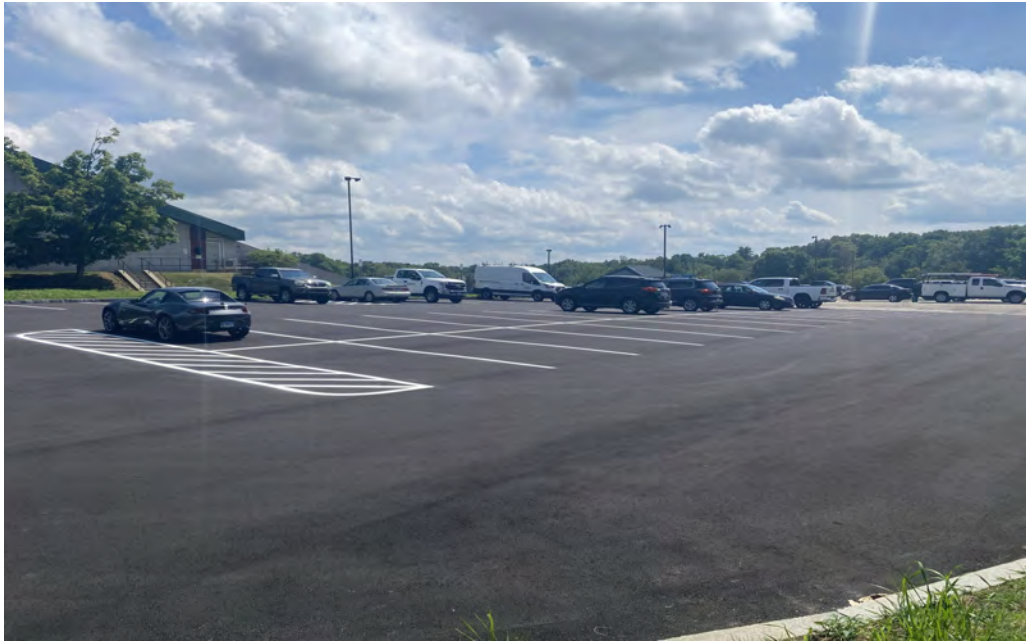
New parking lot from southwest
