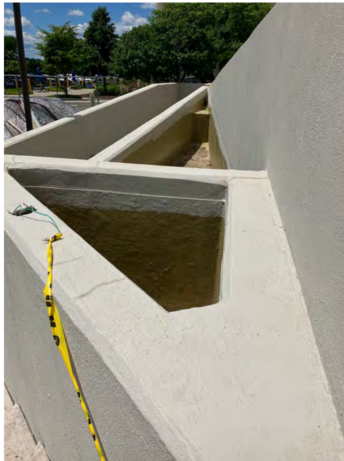
New Bituthene and Kemper Waterproofing at Existing Planters
