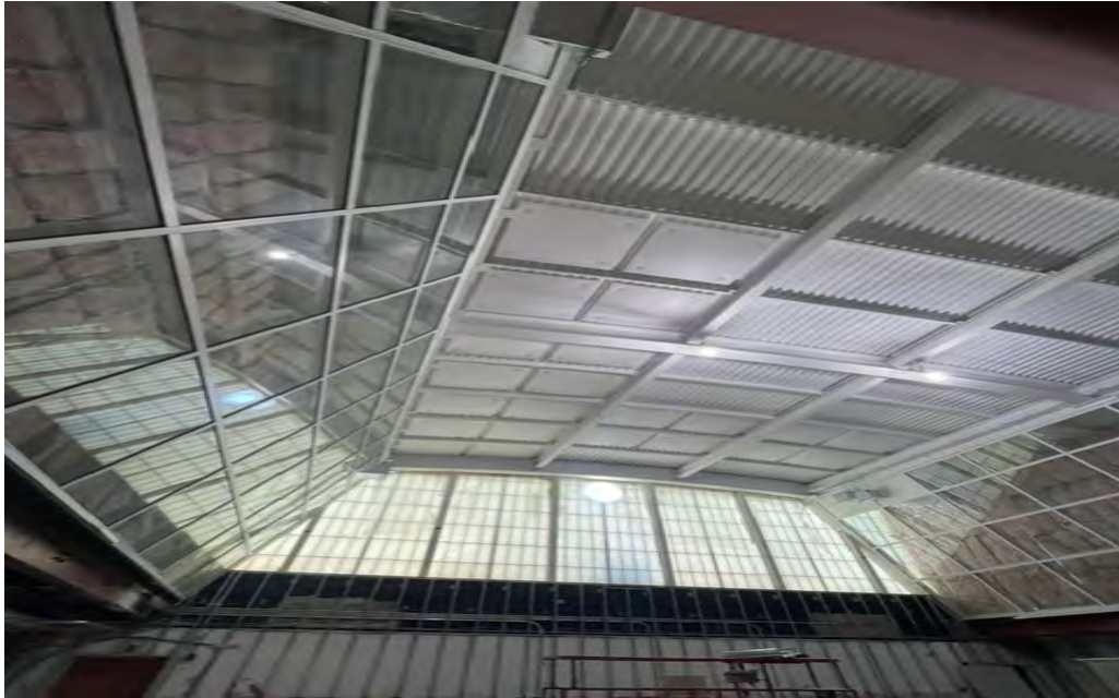
Phase II - Hydro Therapy Area - Acoustical Panels Install
