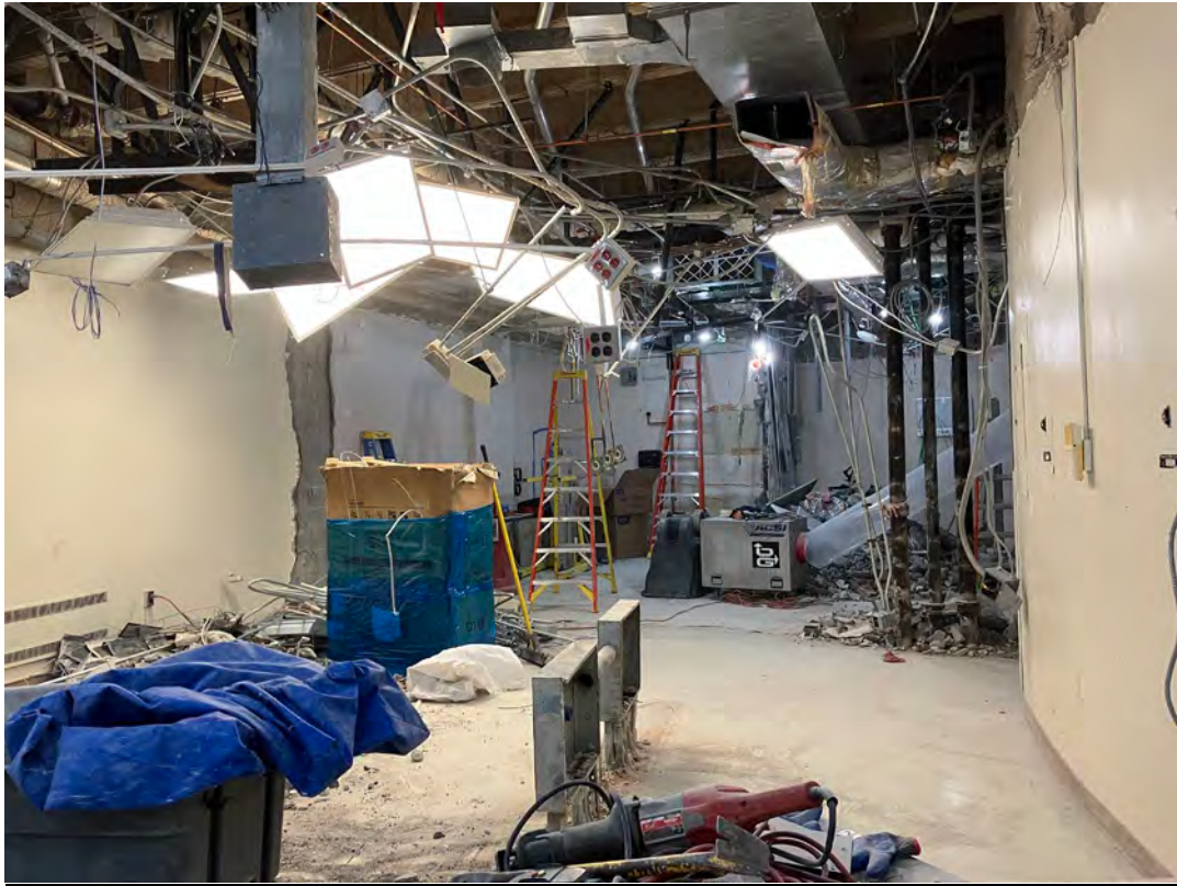
Demo in Progress at Future IR Suite
