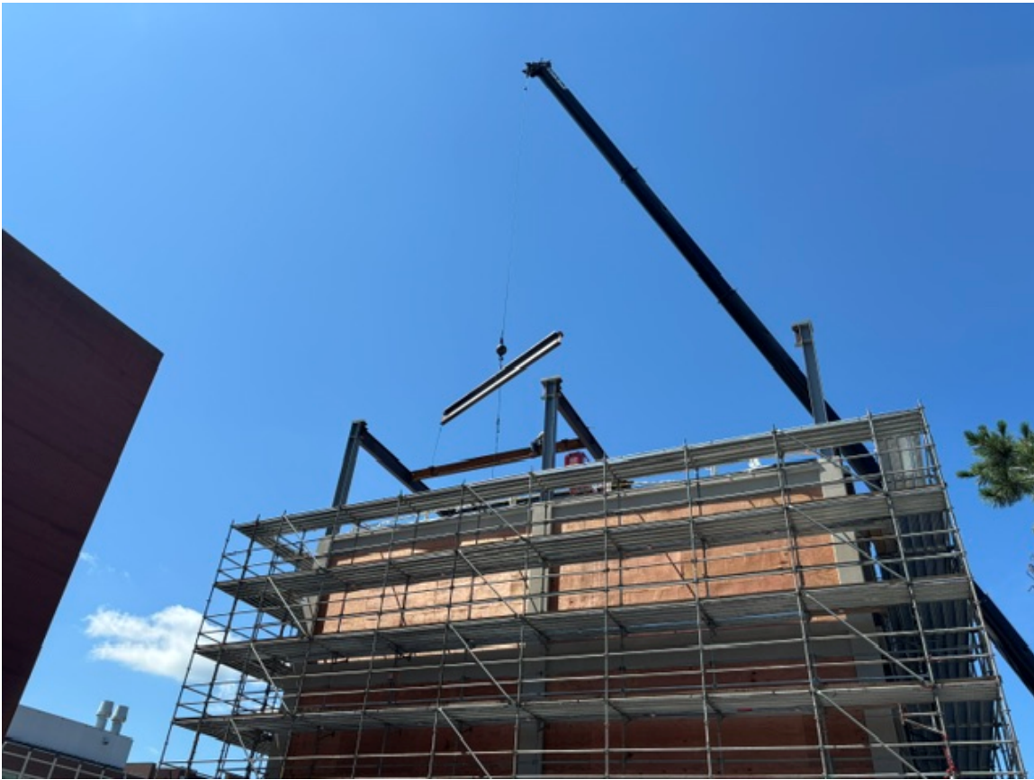
4th Floor Steel Erection
