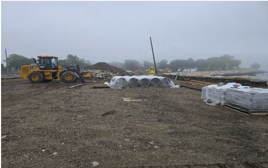
Stormwater materials on Site
