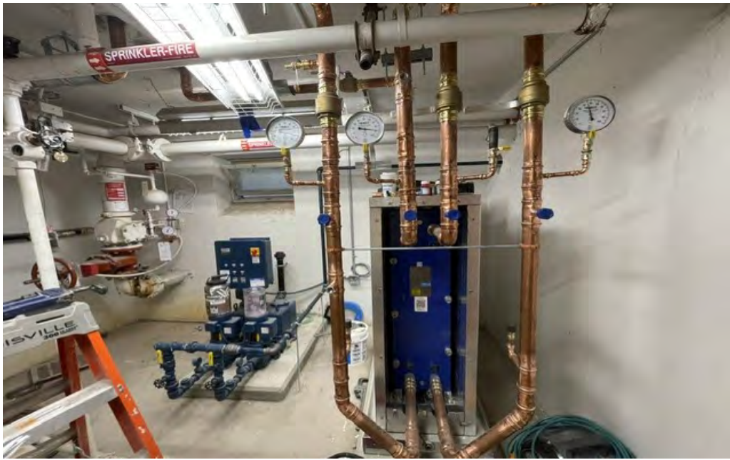
Heat Exchanger Installation Typical
