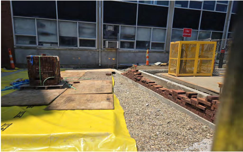
Exterior dumpster slab complete & screen wall underway
