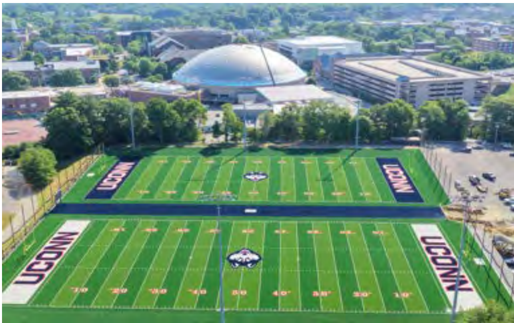
Upgrade entry in progress, scoreboard in place, new fencing
