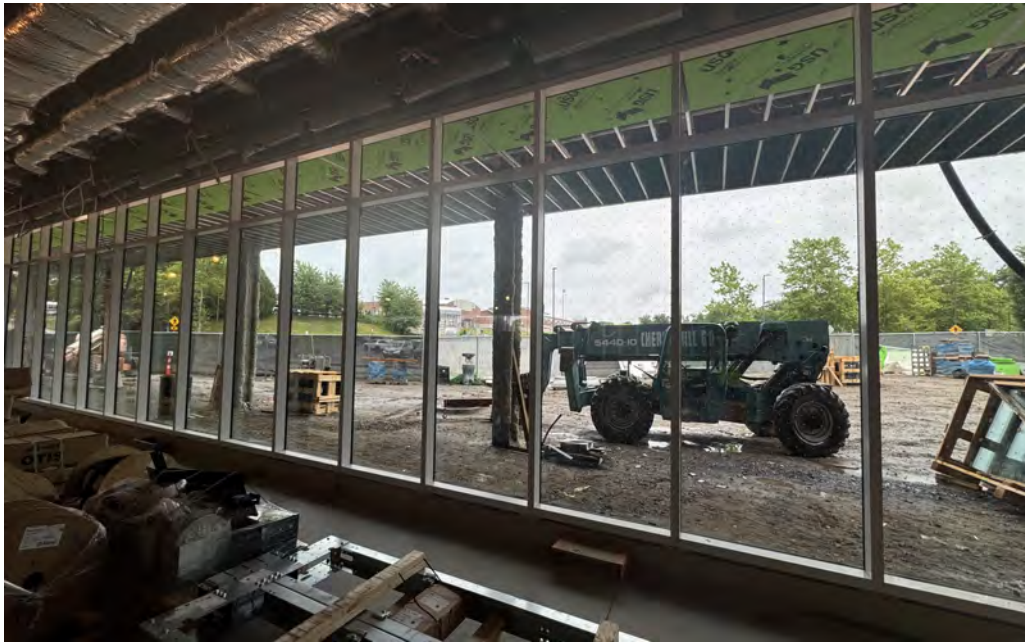
Window framing & glazing install -Level 1 -South Elevation
