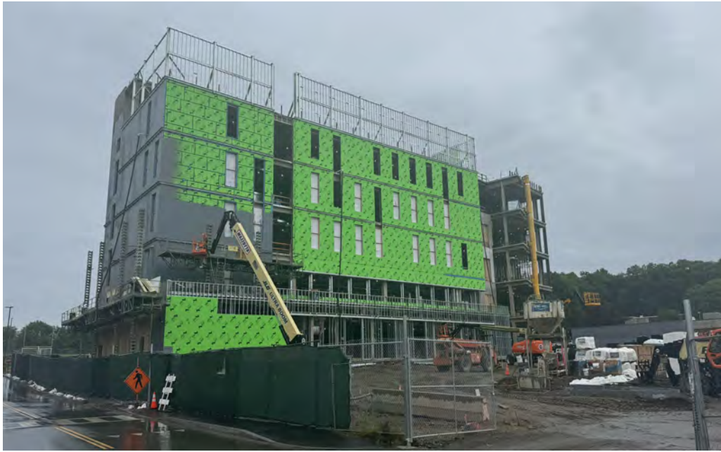
Exterior Facade progress - North Elevation
