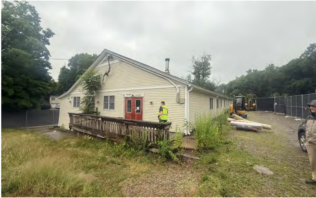
Existing Structure Before Demolition
