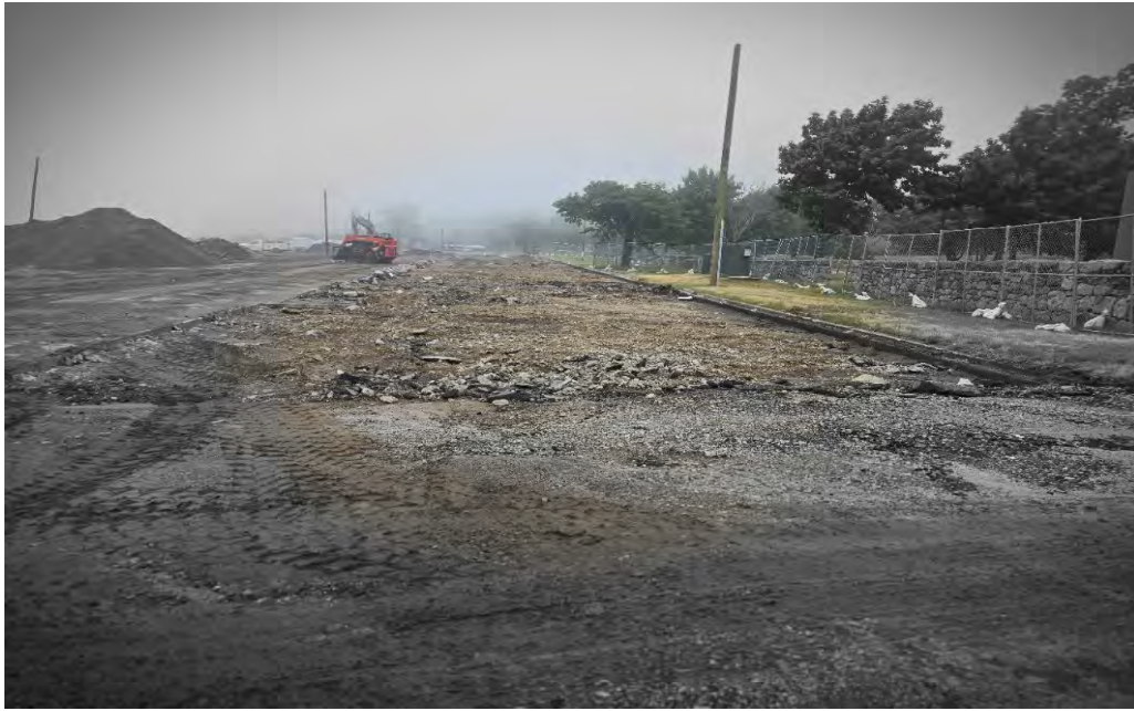
Milling of Existing Pavement is complete
