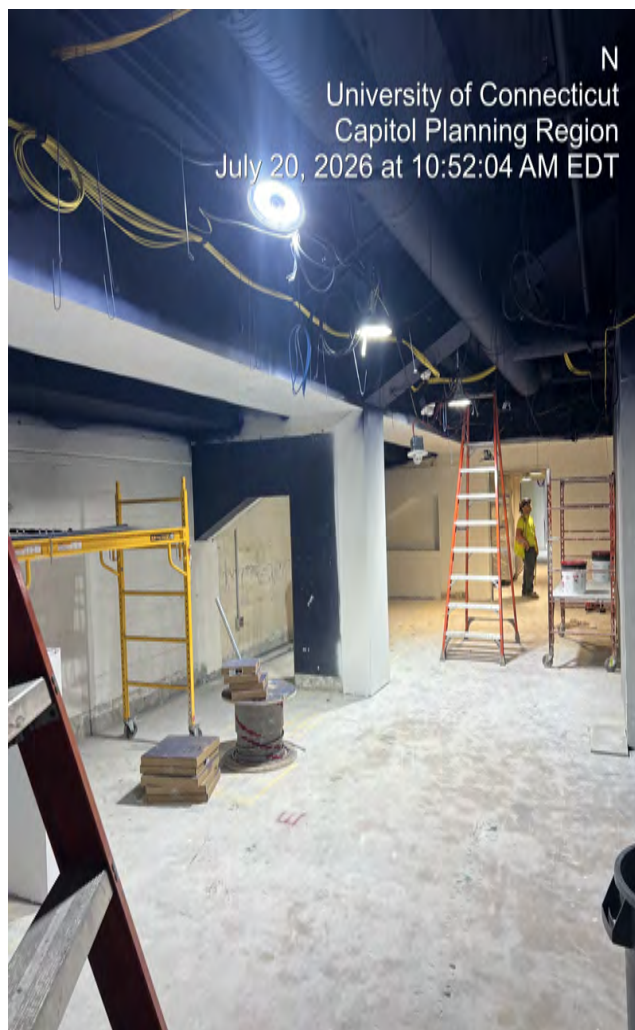
Grab and Go Renovations
